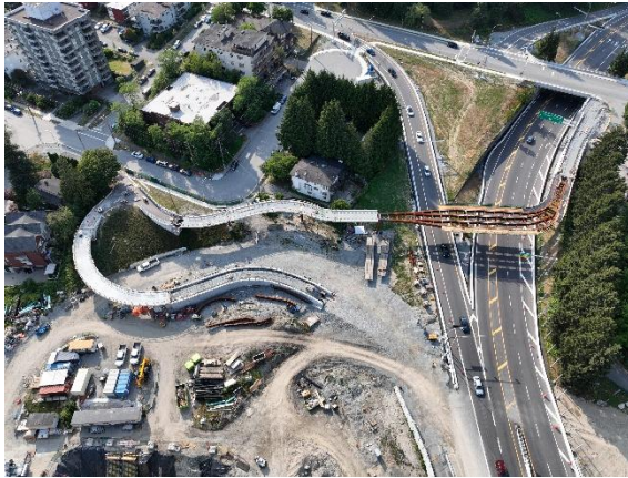
Figure 1: The Agnes Royal Multi-use Path overpass progress.
