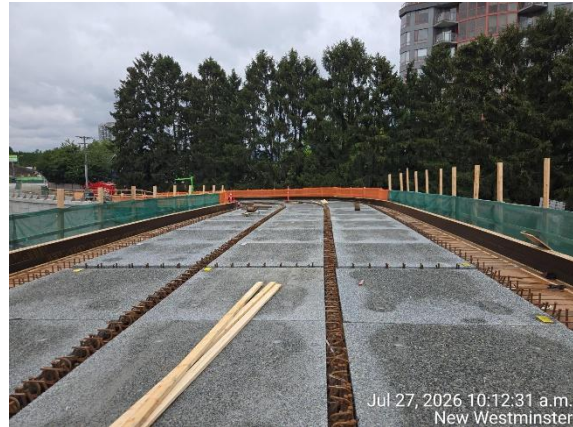
Figure 2: Concrete deck panels installed on the Royal Agnes Multi-use path overpass.
