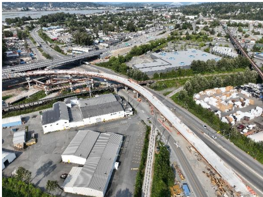
Figure 3: Highway 17 off-ramp and multi-use path progress.
