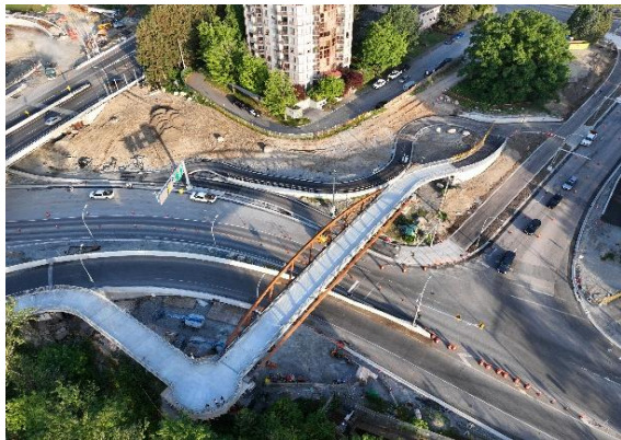
Figure 3: Completed Columbia multi-use path overpass in New Westminster.
