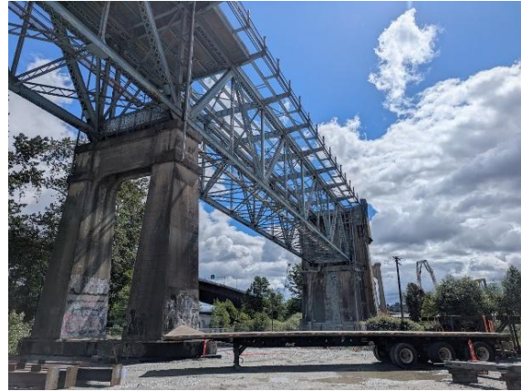
Figure 2: Deconstruction progress of the Pattullo Bridge in Surrey.
