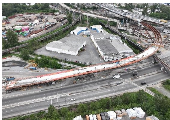
Figure 4: Highway 17 off-ramp progress.
