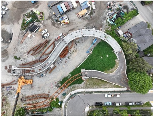
Figure 1: Construction progress on the multi-use path structures in New Westminster.
