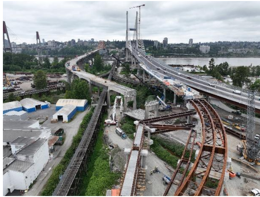
Figure 2: Deconstruction of the Pattullo Bridge south approach in Surrey, and Highway 17 off-ramp progress.
