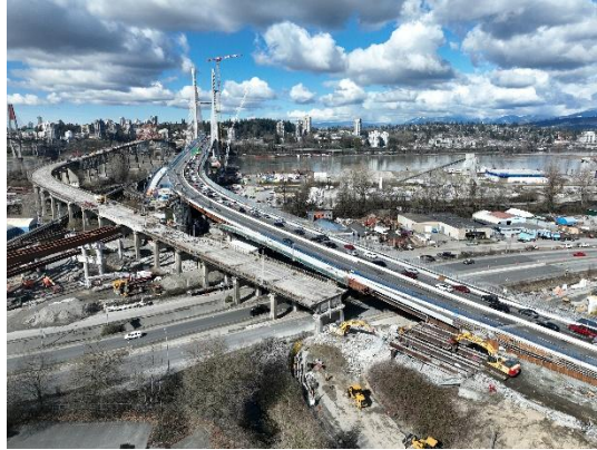
Figure 2: Deconstruction of the Pattullo Bridge south approach in Surrey.
