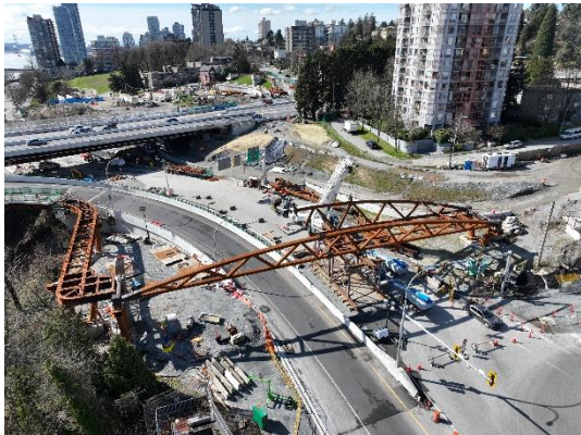
Figure 3: Construction progress on the Columbia multi-use path overpass in New Westminster.
