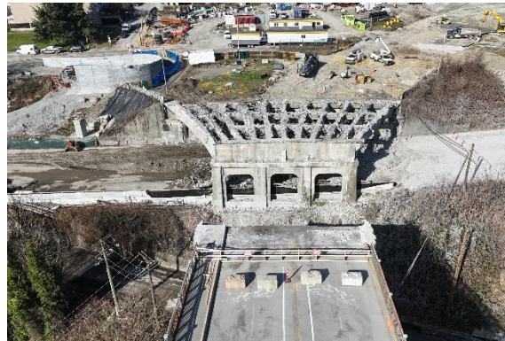
Figure 4: Deconstruction of the Pattullo Bridge north approach in New Westminster.
