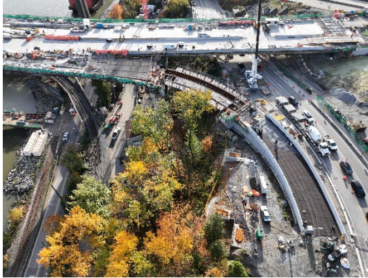
Figure 1: New Westminster - East Columbia Exit Ramp paving underway.
