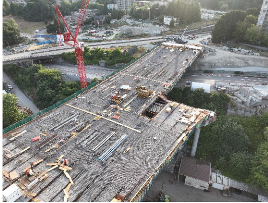
Figure 1: North Approach in New Westminster - Crews continue deck panel and rebar installation and prepare for deck concrete pours.
