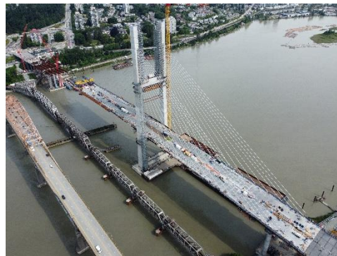
Figure 4: Bridge finishing activities underway on the main span.
