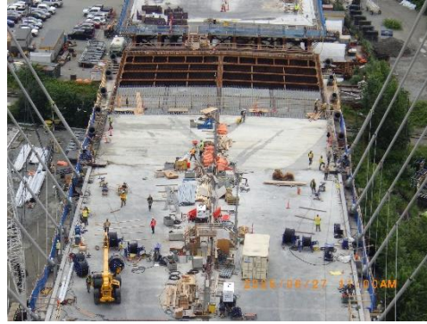
Figure 2: Concrete deck overlay pour preparation for the end span on the bridge.
