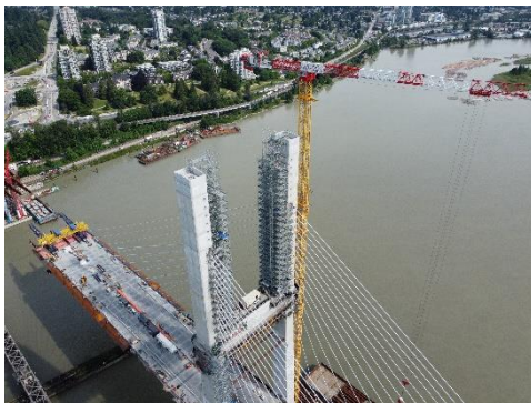
Figure 3: Stay cable installation continues.
