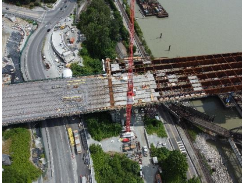
Figure 1: Steel bracing and precast deck panel installation continues on the north approach in New Westminster.
