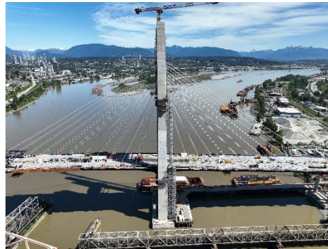
Figure 4: Main bridge tower, main span and back span, showing stay cable progress.
