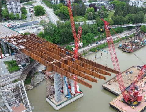
Figure 1: Steel girder erection for North Approach in New Westminster completed.
