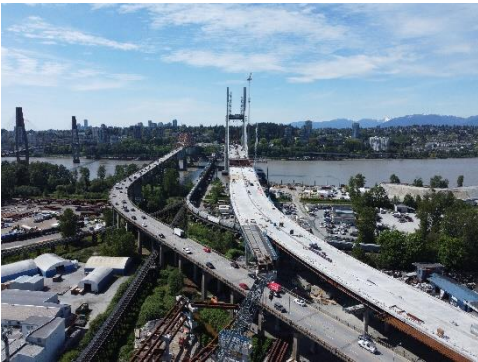
Figure 3: View of the South Approach showing the new off-ramp under construction which will connect southbound vehicles directly to Highway 17 westbound.
