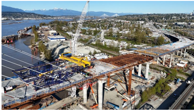
Figure 1: Connection completed between the back span to the end span and south approach.
