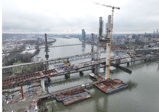
Figure 2: Main span is advancing with deck panel installation and preparations for steel girder connection of the back span to the end span.
