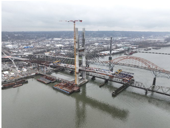
Figure 3: Girder erection, deck panel, and stay cable installation for the main bridge continues. In this photo, 18 of 40 cables stays have been installed.
