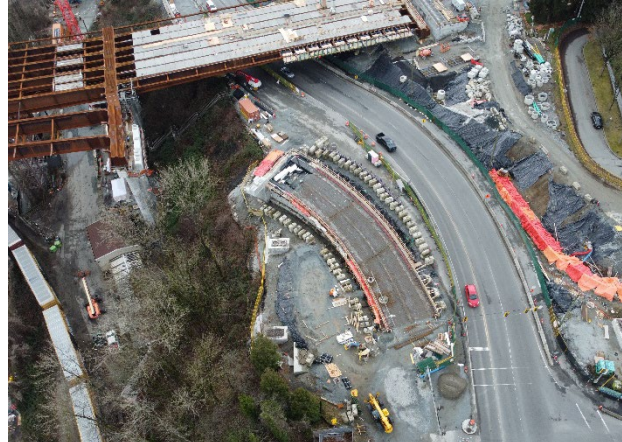
Figure 2: Construction of the new direct E. Columbia Street off-ramp is ongoing.
