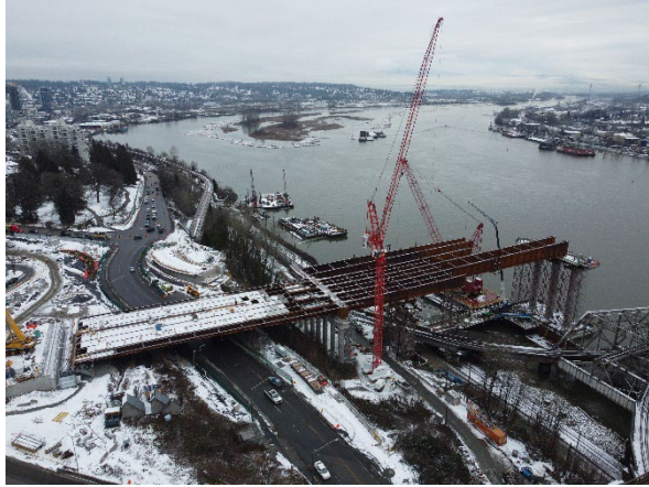
Figure 1: North Approach girder erection continues in New Westminster.
