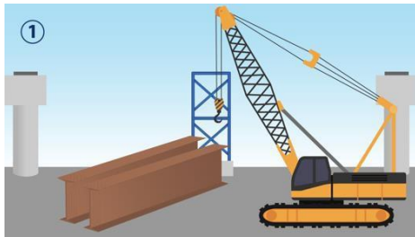
1. A large crane lifts the steel girder.
