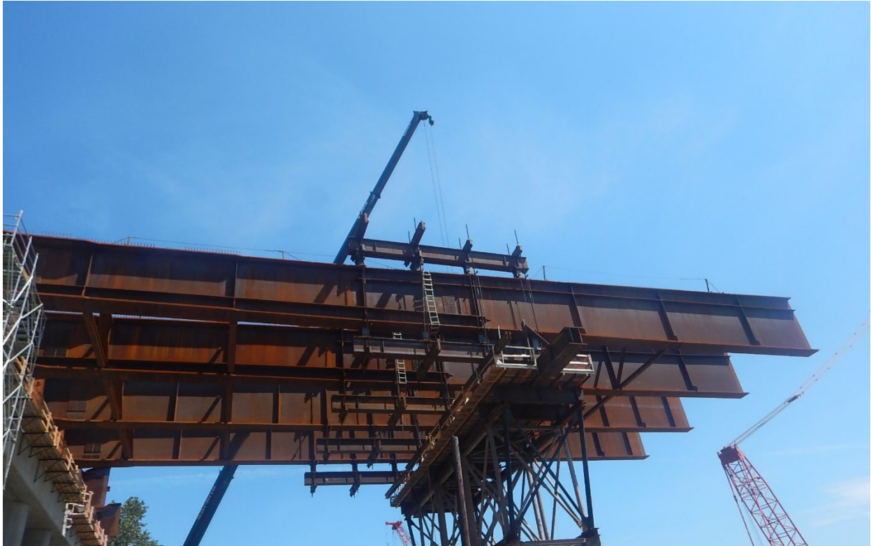
Figure 3 – North Approach girder erection continued above Front Street in New Westminster.
