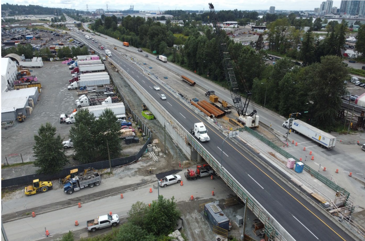
Figure 1 – In Surrey, Highway 17 eastbound traffic was moved onto the completed portion of the Old Yale Road Overpass. Crews have started construction of the westbound portion of the Old Yale Road Overpass.
