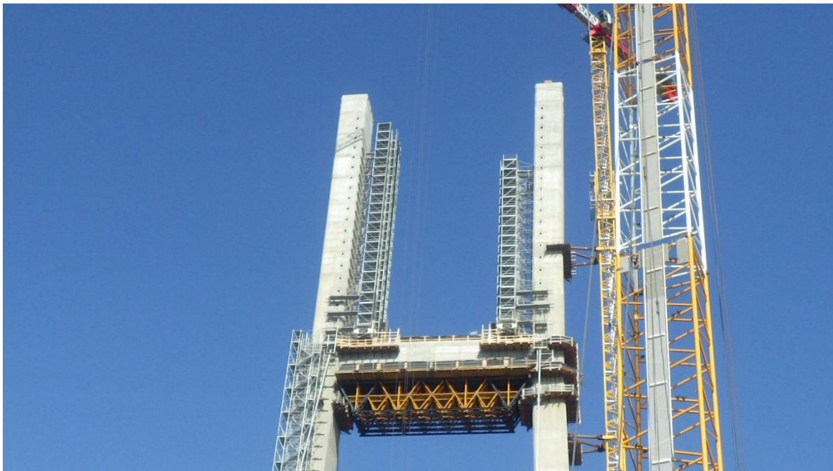
Figure 2 – Tower construction formwork was removed from both legs.
