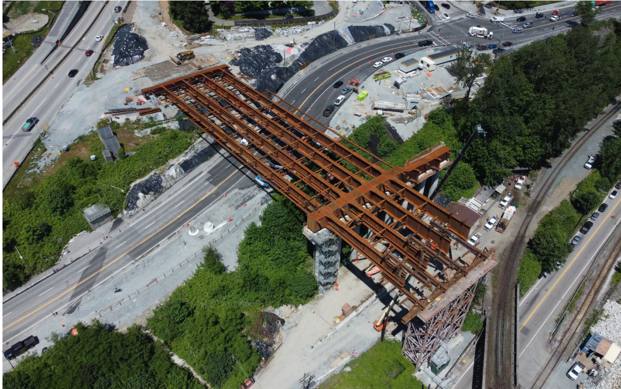
Figure 3 – Aerial of the completed north approach girder erection over Columbia Street in New Westminster.
