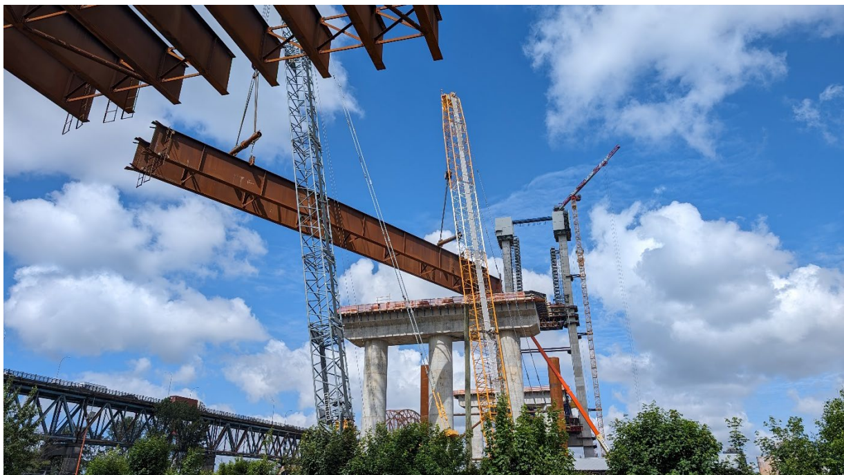
Figure 2 – A paired girder being erected at the south approach in Surrey.
