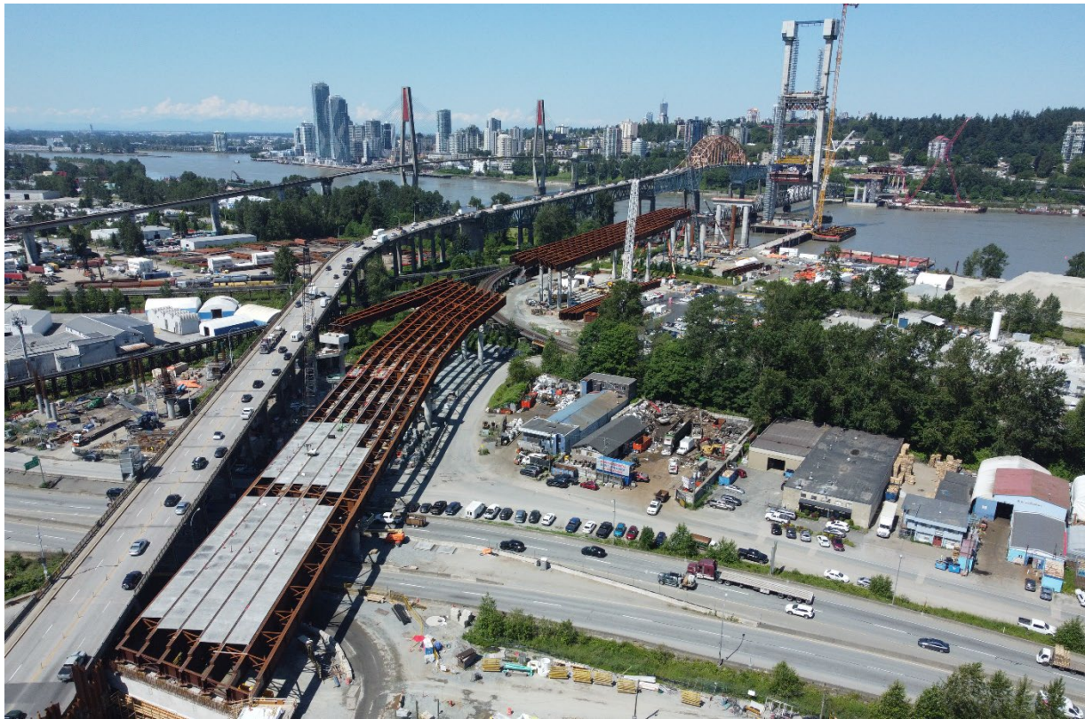
Figure 1 – In Surrey, crews have begun installing precast deck panels onto the south approach girders.
