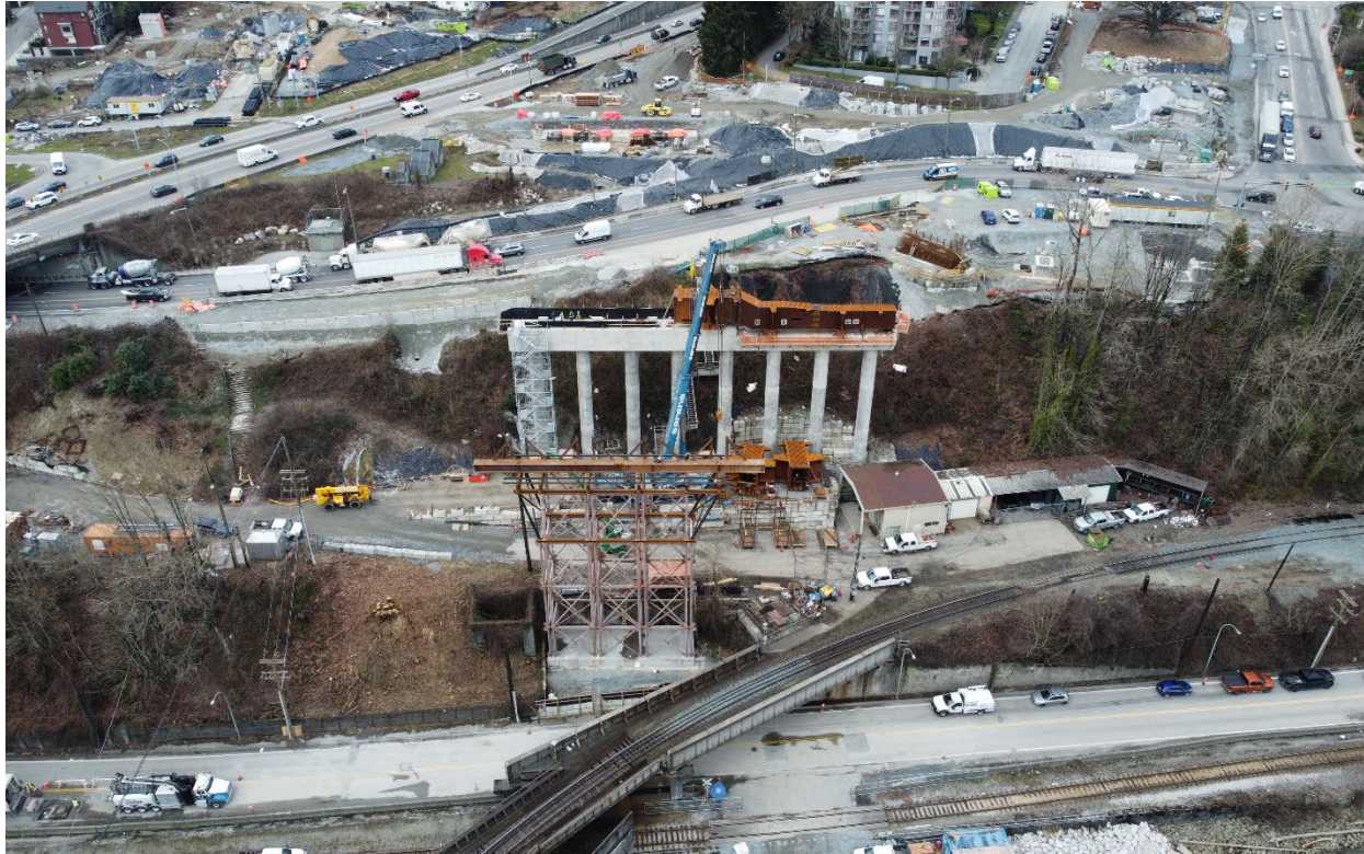
Figure 3 – Aerial of pier N2 in New Westminster during preparation for girder installation.
