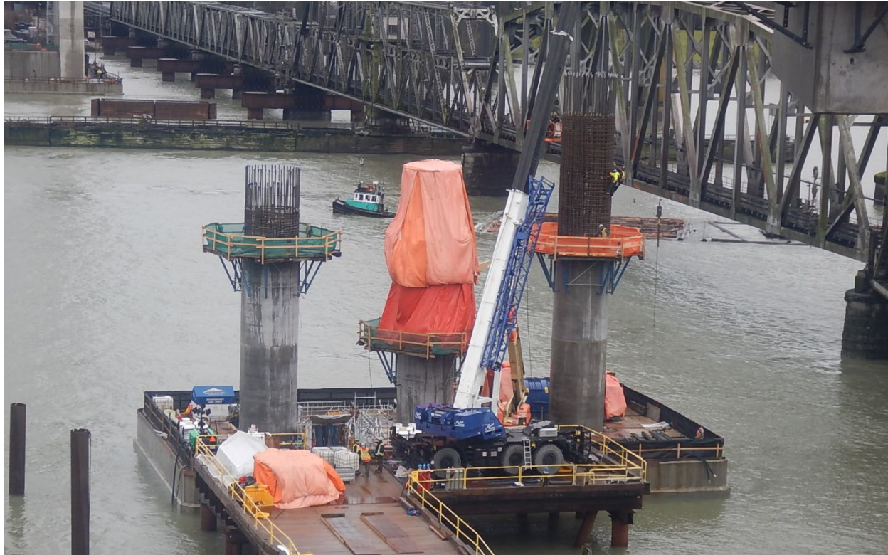
Figure 3 – Ongoing construction of Pier N1 columns
