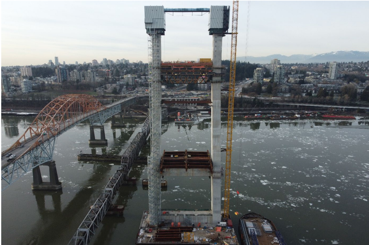
Figure 1 – Aerial of ongoing main bridge tower and pier table construction
