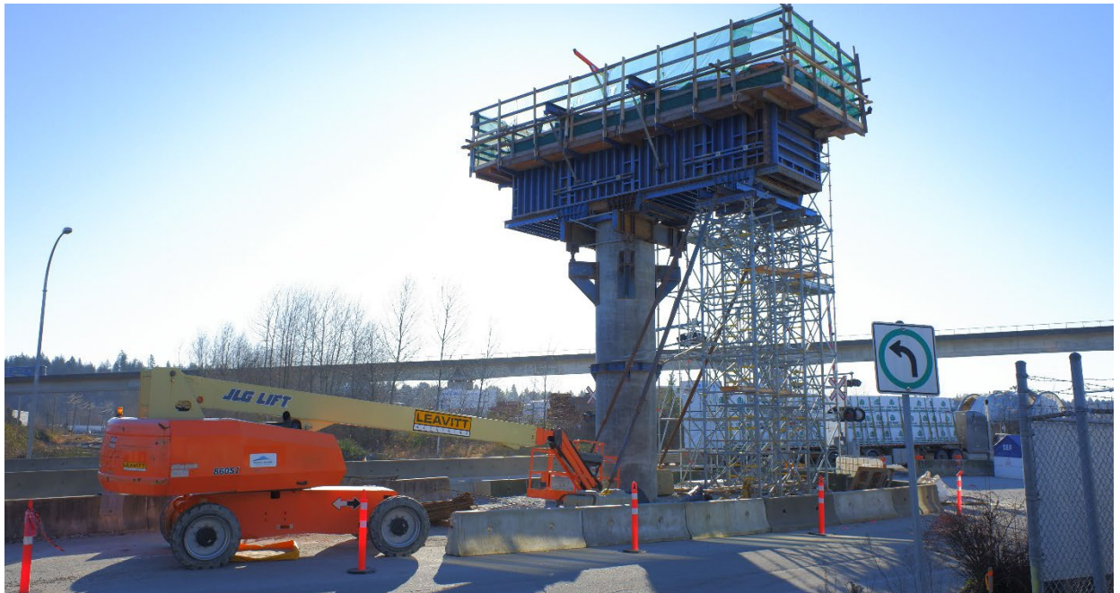
Figure 4 – Ongoing construction of SR4 pier cap
