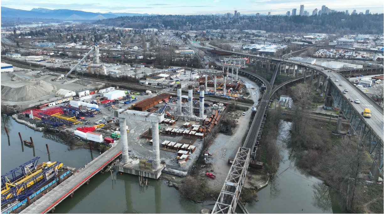
Figure 3: Aerial of the Surrey site showing Pier S2 to the south abutment.
