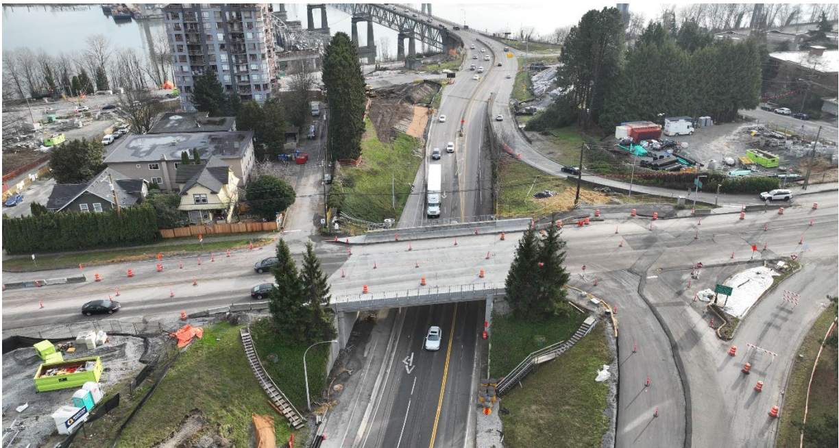
Figure 4: Aerial of ongoing rehabilitation work on Royal Avenue.
