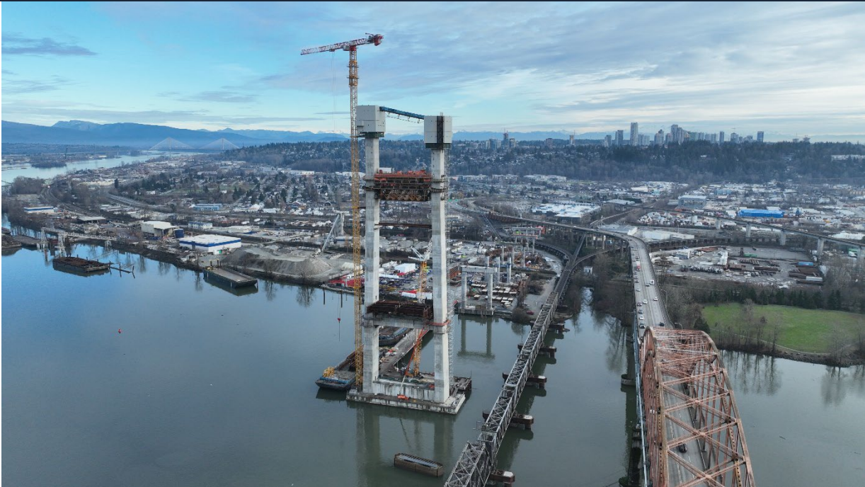
Figure 1 – Aerial of ongoing Pier S1 Tower Construction
