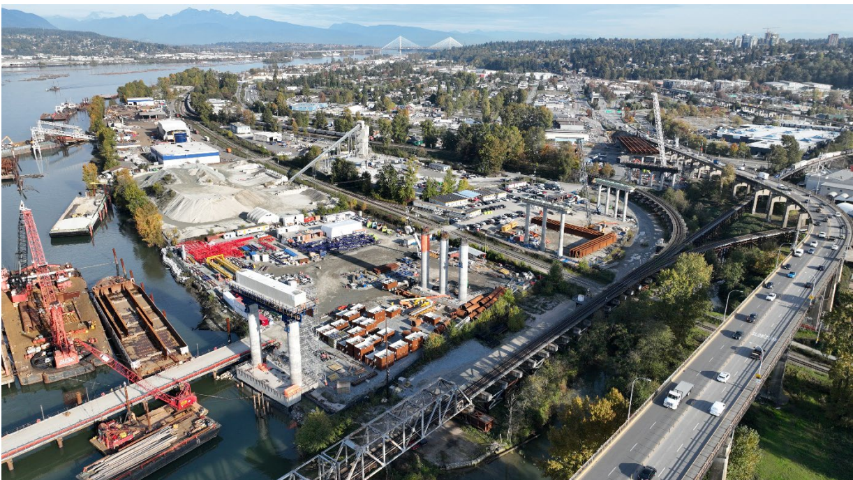
Figure 2 – Aerial of the Surrey site showing pier S2 to the south abutment.
