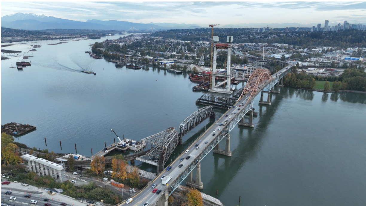
Figure 3: Aerial of the Pattullo Bridge Replacement Project in the Fraser River
