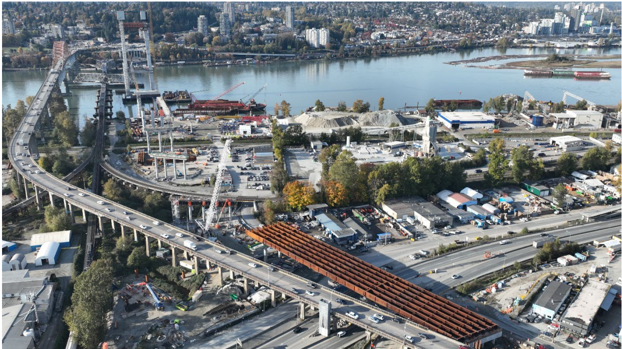
Figure 3 – Girder Construction In Surrey From South Abutment To Pier S7
