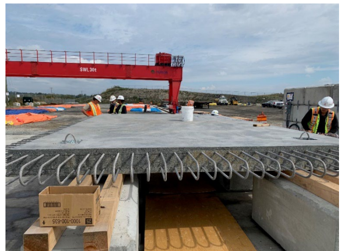
Concrete has cured and the deck panel has been stripped.
