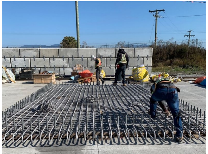
Deck panel formwork is constructed before concrete is poured.
