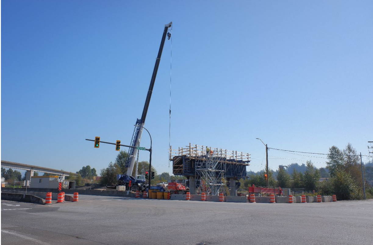
FIGURE 3 – CONSTRUCTION CONTINUES ON THE NEW GRADE SEPERATED OLD YALE ROAD OVERPASS
