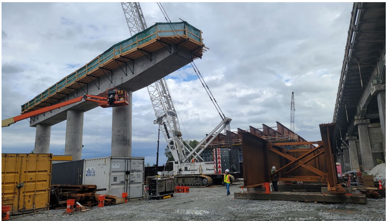
FIGURE 2 – GIRDER CONSTRUCTION IN SURREY CONTINUES FROM S7 TO S8
