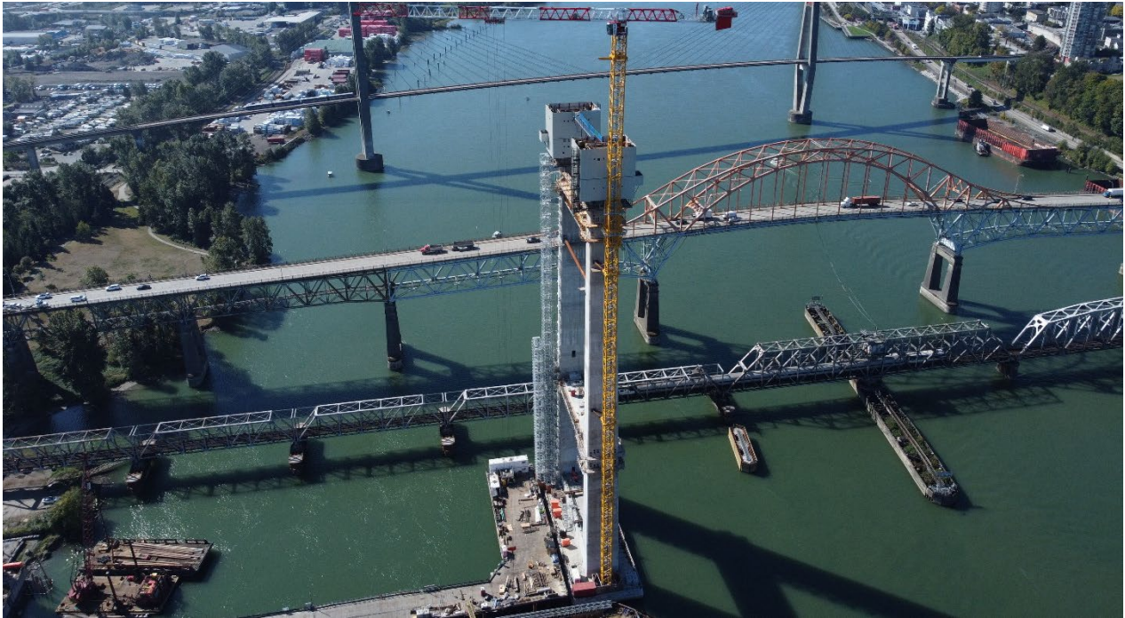
FIGURE 1 – AERIAL OF ONGOING S1 TOWER CONSTRUCTION
