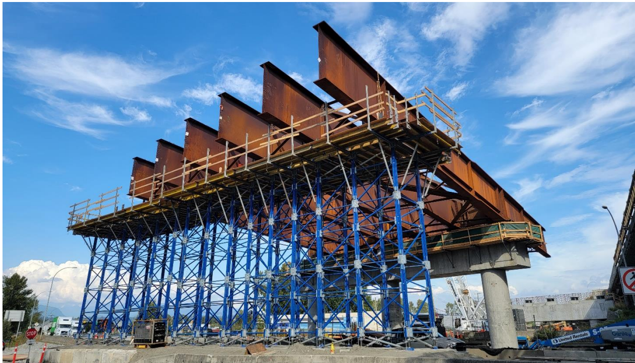
FIGURE 2 – PHOTO OF THE GIRDER CONSTRUCTION OVER HIGHWAY 17 WHICH BEGAN IN AUGUST
