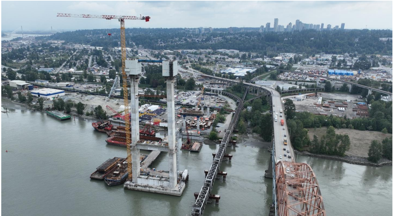
FIGURE 1 – AERIAL OF ONGOING S1 TOWER CONSTRUCTION, LOOKING SOUTH
