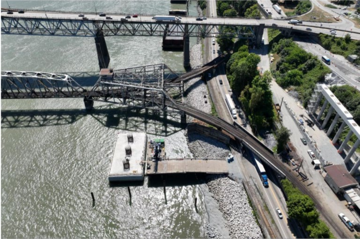
FIGURE 3 – AERIAL OF THE 27-HOUR N1 PILE CAP CONCRETE POUR
