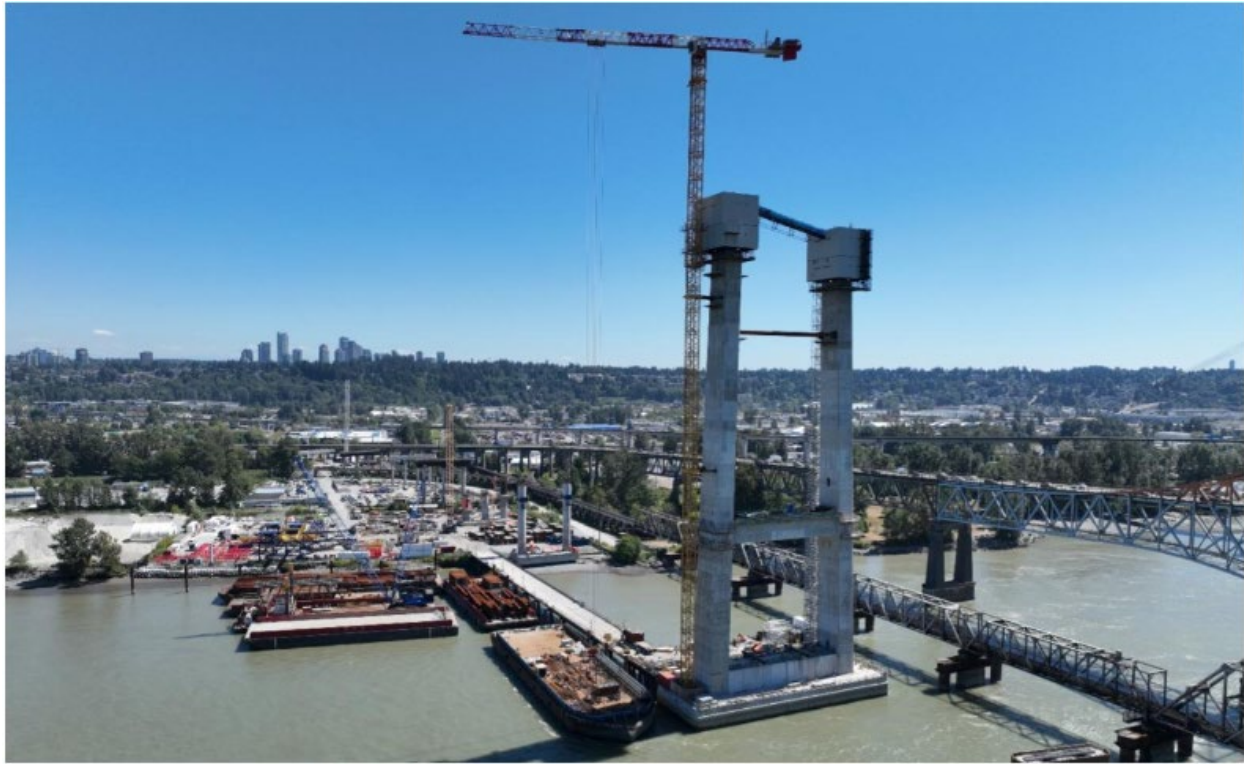
FIGURE 1 – AERIAL OF ONGOING S1 TOWER AND CROSSBEAM CONSTRUCTION, LOOKING SOUTH
