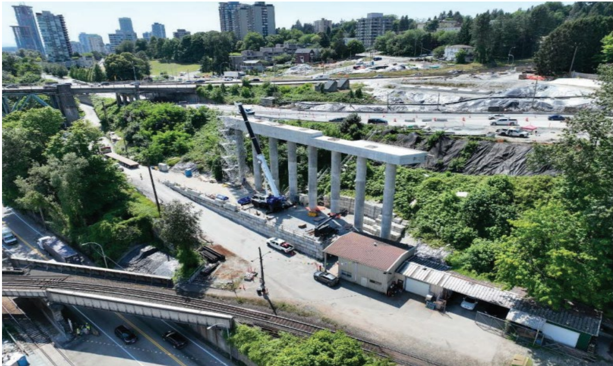
FIGURE 4 – AERIAL OF THE ONGOING WORK AT N2
