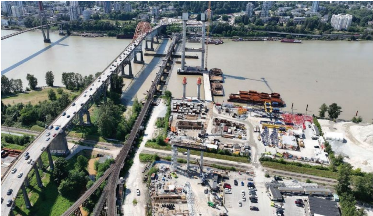
FIGURE 2 – AERIAL OF THE ONGOING S2 COLUMN CONSTRUCTION AND S3 PIER CAP CONSTRUCTION
