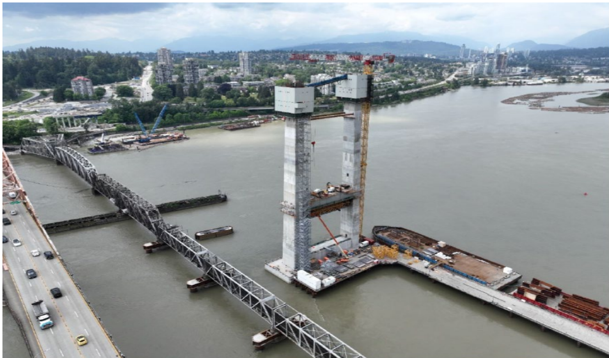
FIGURE 2 – AERIAL OF THE ONGOING S1 TOWER AND CROSSBEAM CONSTRUCTION, LOOKING NORTHEAST
