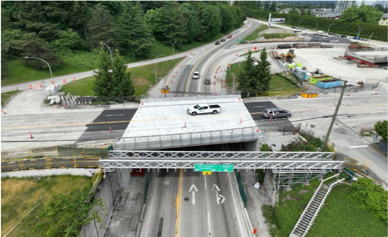
FIGURE 4 – AERIAL OF THE COMPLETED ROYAL AVENUE OVERPASS DECK REPLACEMENT
