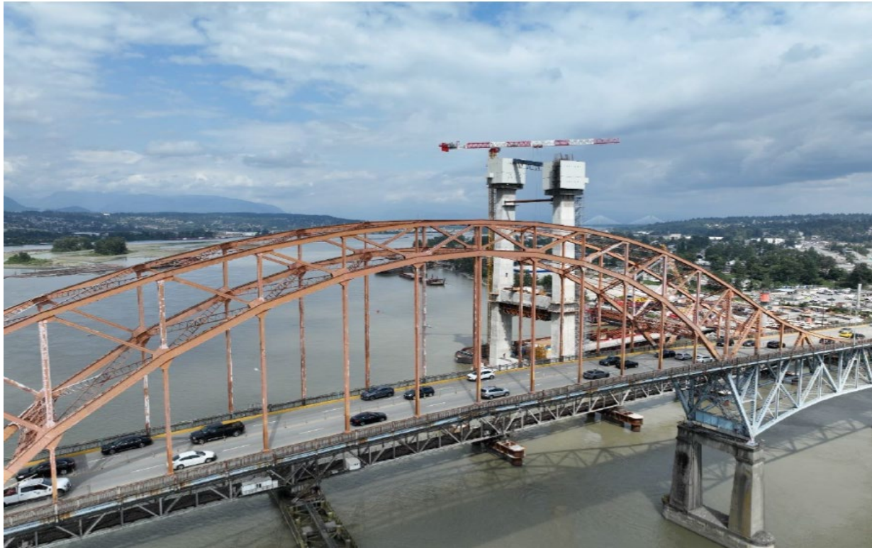
FIGURE 1 – AERIAL OF THE ONGOING S1 TOWER CONSTRUCTION, LOOKING EAST
