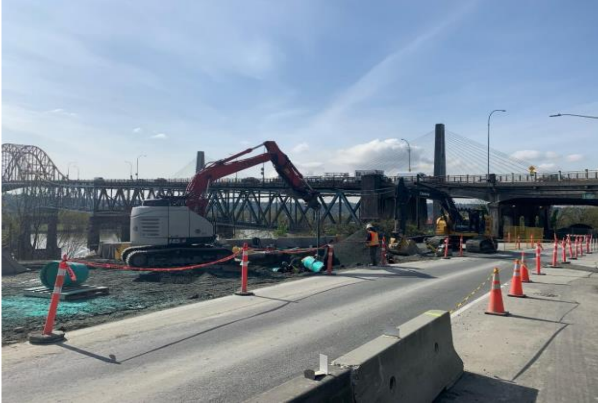
FIGURE 3 – PHOTO TAKEN OF THE ONGOING COLUMBIA STREET UTILITY WORK
