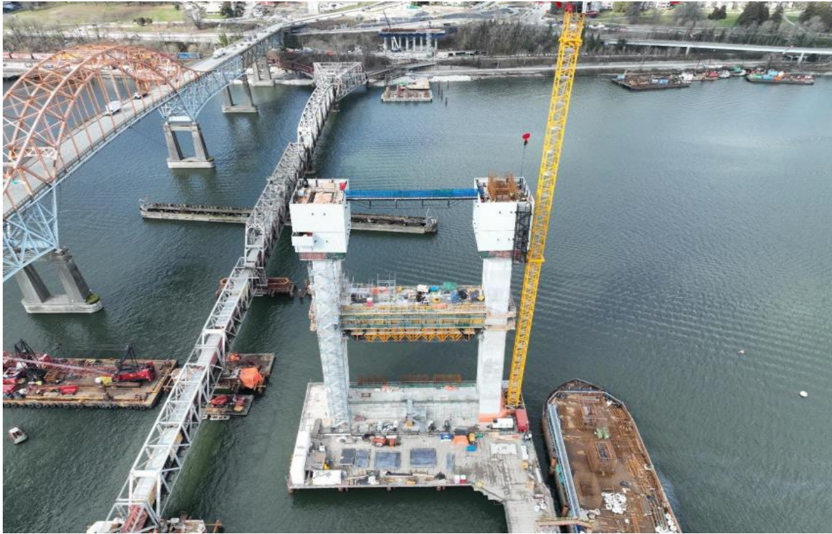
FIGURE 1 - AERIAL OF ONGOING S1 TOWER AND CROSSBEAM CONSTRUCTION, LOOKING SOUTHWEST
