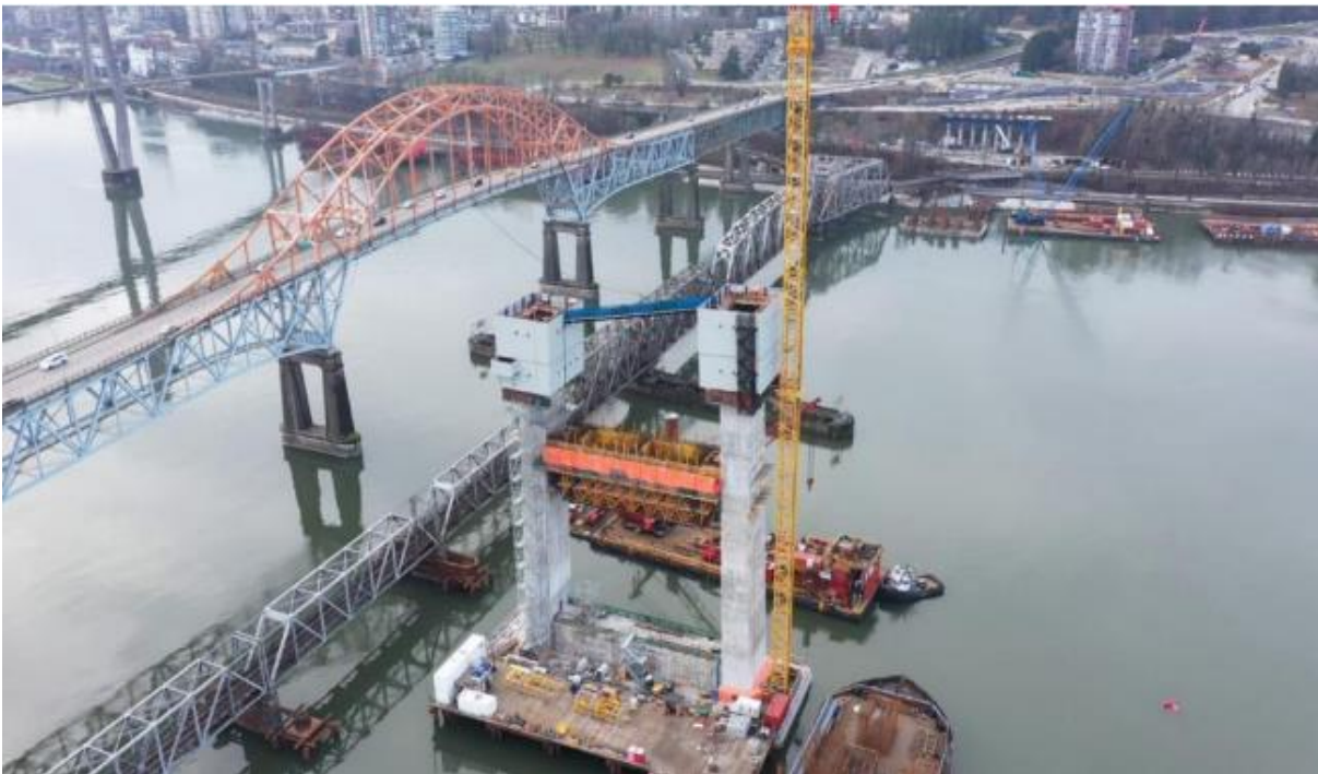
FIGURE 2 – AERIAL OF S2 AND S4 COLUMN CONSTRUCTION
