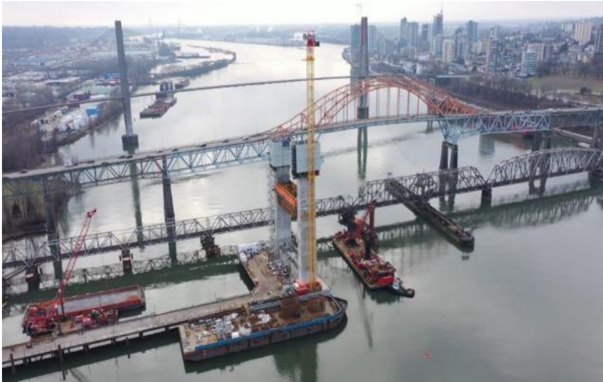
FIGURE 3 – AERIAL OF S4 COLUMN CONSTRUCTION AND S5 PIER CAP CONSTRUCTION
