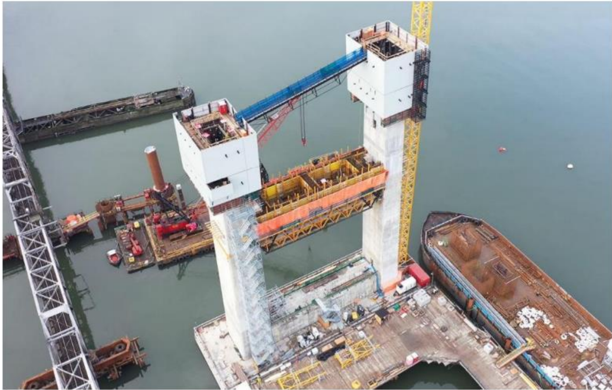
FIGURE 1 – AERIAL OF THE S1 TOWER AND CROSSBEAM CONSTRUCTION, LOOKING SOUTH
