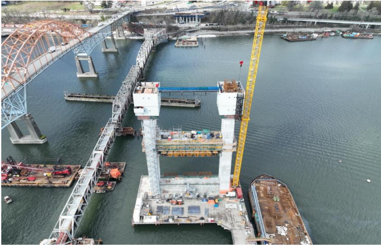
FIGURE 1 - AERIAL OF THE S1 TOWER AND CROSSBEAM CONSTRUCTION, LOOKING NORTH
