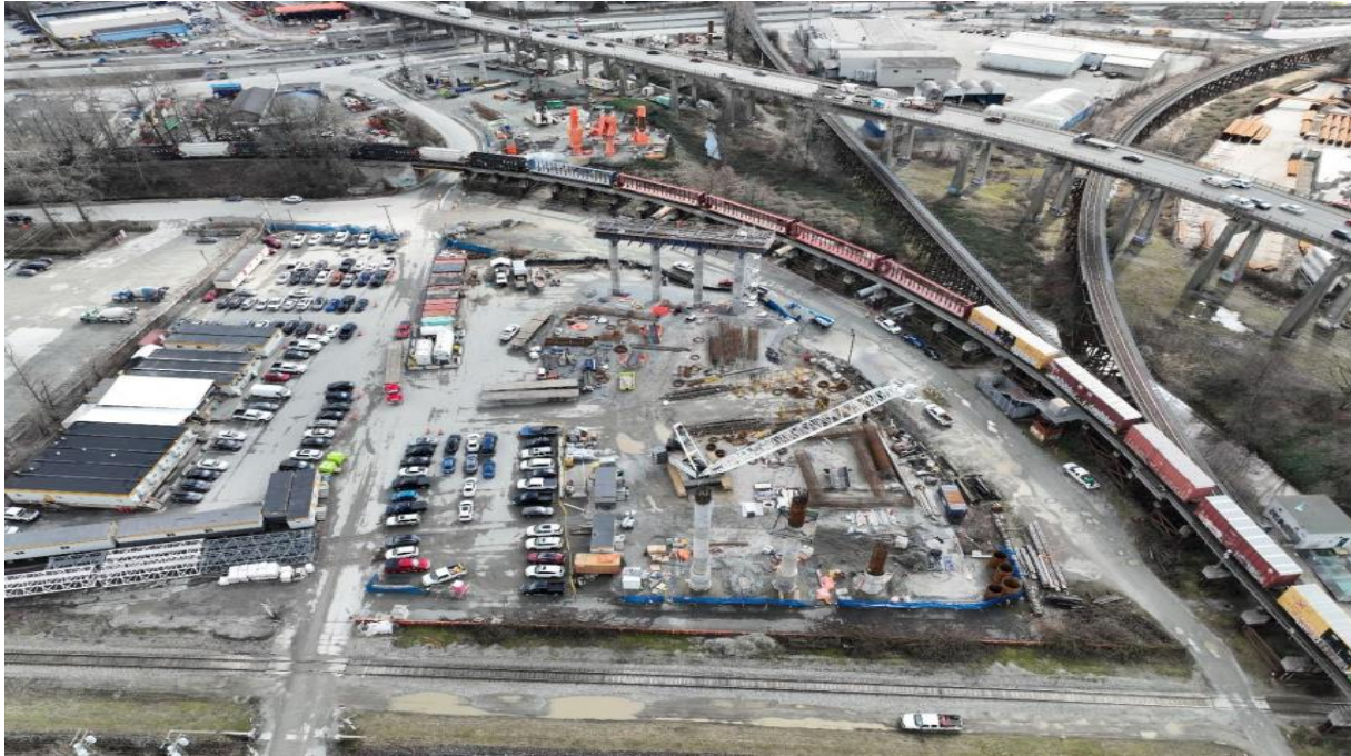
FIGURE 3 – AERIAL OF THE S4 COLUMN CONSTRUCTION AND S5 PIER CAP CONSTRUCTION
