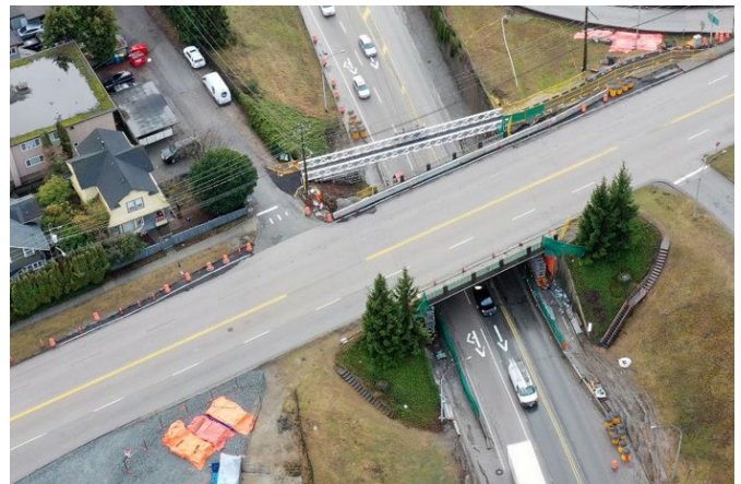
Royal Avenue overpass crossing over the Bridge Connector
