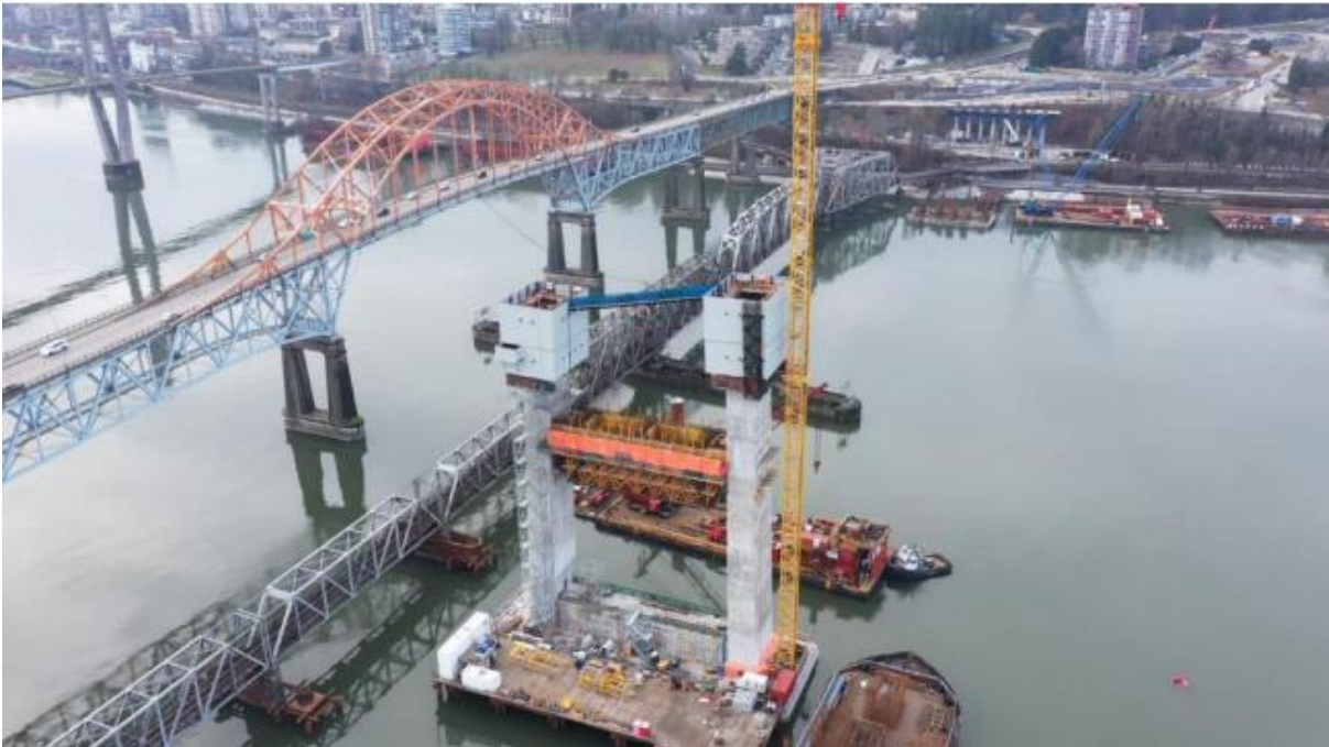
FIGURE 2 – AERIAL OF THE S1 TOWER AND CROSSBEAM CONSTRUCTION, LOOKING NORTH
