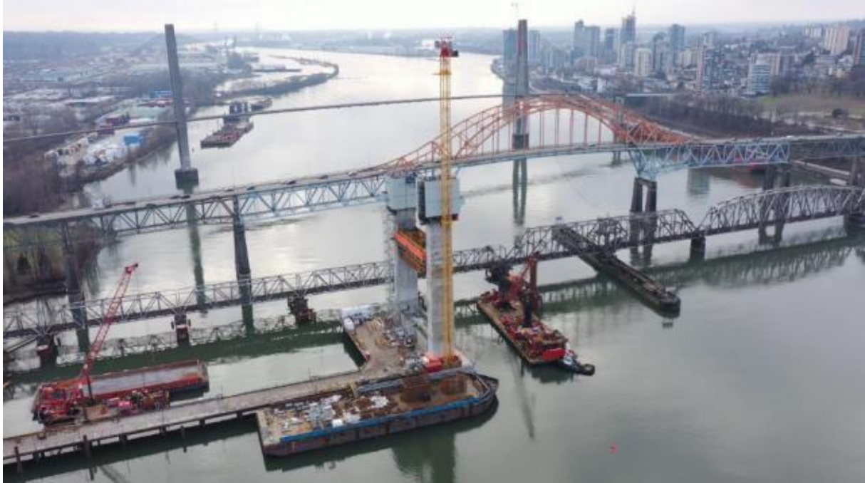
FIGURE 3 – AERIAL OF THE S1 TOWER AND CROSSBEAM CONSTRUCTION, LOOKING WEST
