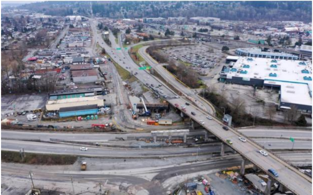
FIGURE 4 – AERIAL OF S8 PIER CAP AND SOUTH ABUTMENT CONSTRUCTION, LOOKING SOUTH
