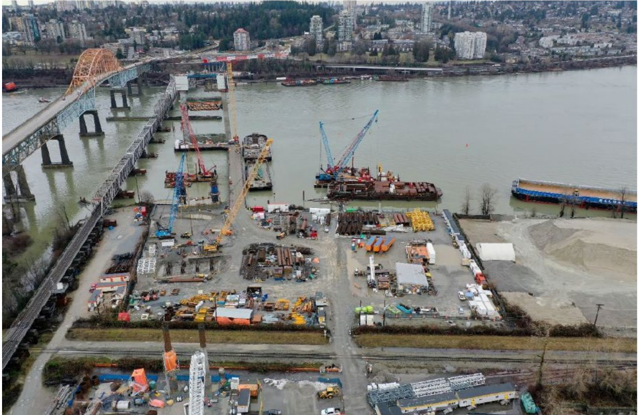
FIGURE 4 – AERIAL OF PIERS S4 TO S1, LOOKING NORTH
