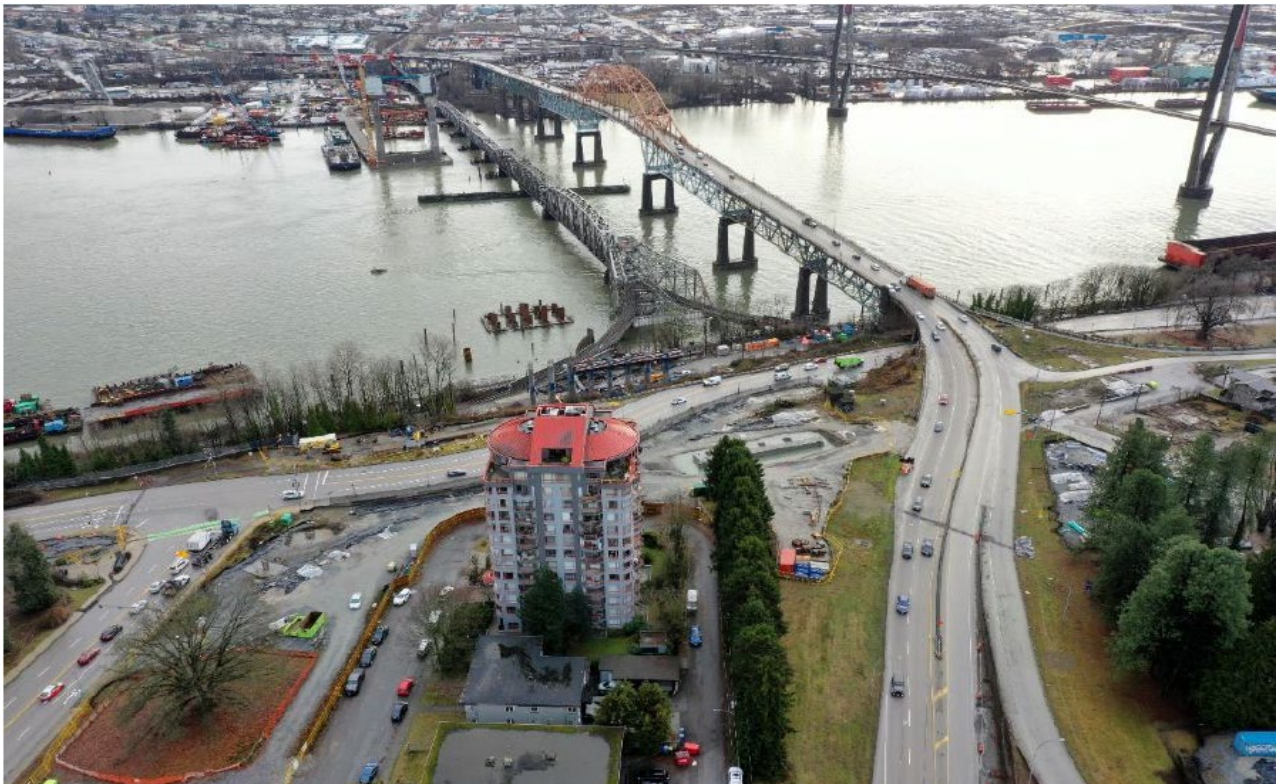
FIGURE 2 – AERIAL OF THE NORTH APPROACH, LOOKING SOUTH
