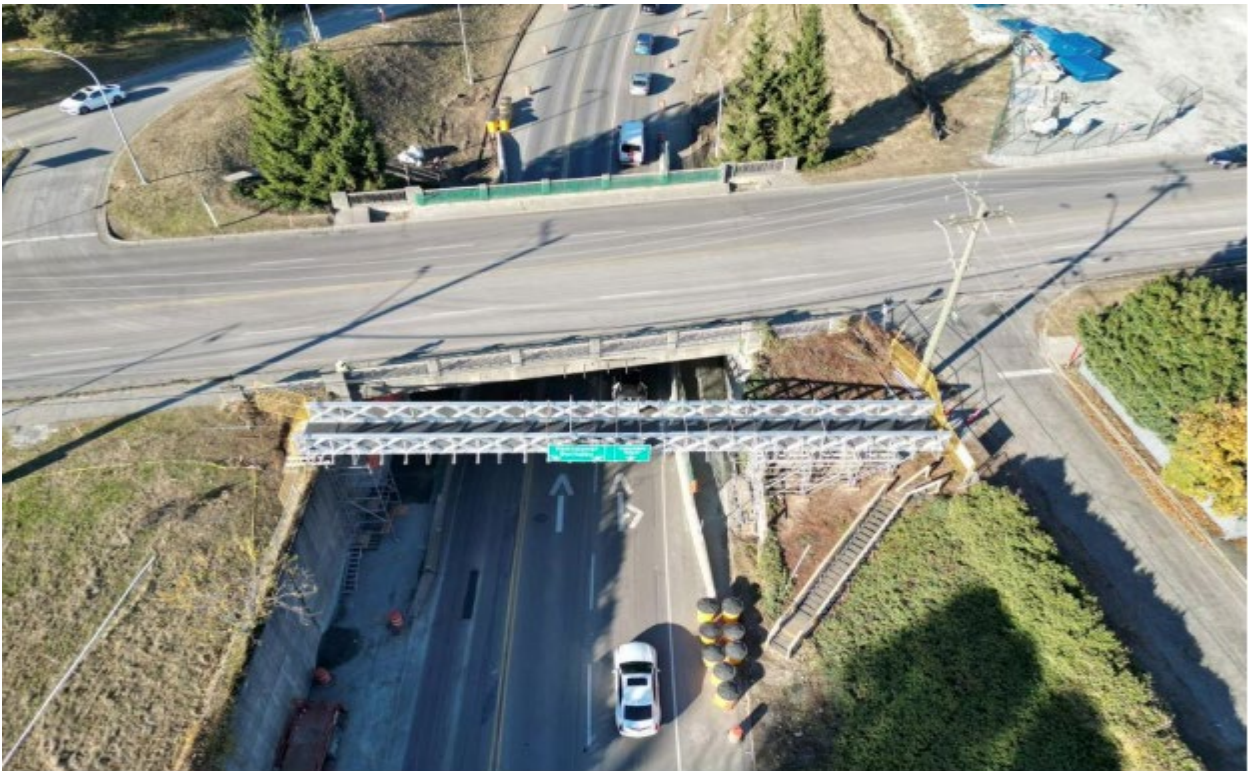
FIGURE 1 – TEMPORARY PEDESTRIAN BRIDGE ACROSS THE ROYAL AVENUE OVERPASS
