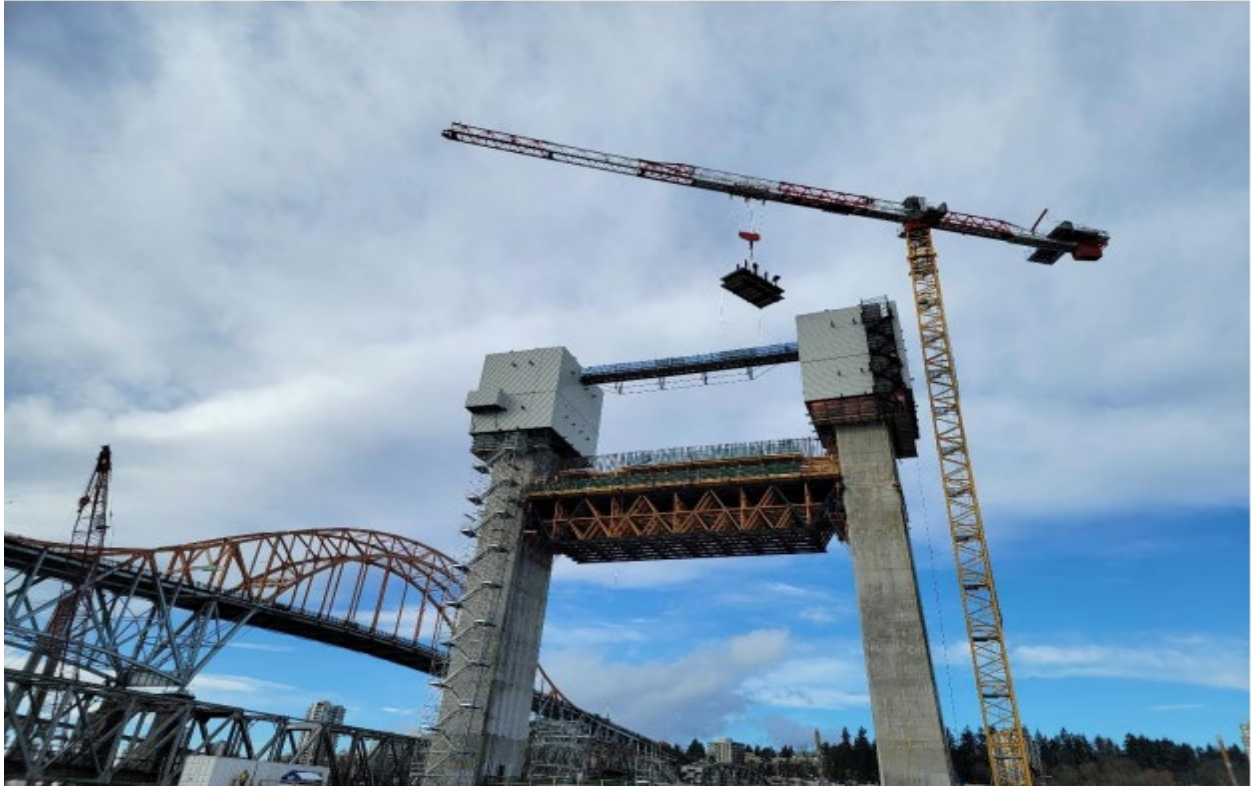
FIGURE 4 – S1 TOWER CROSS BEAM WORK
