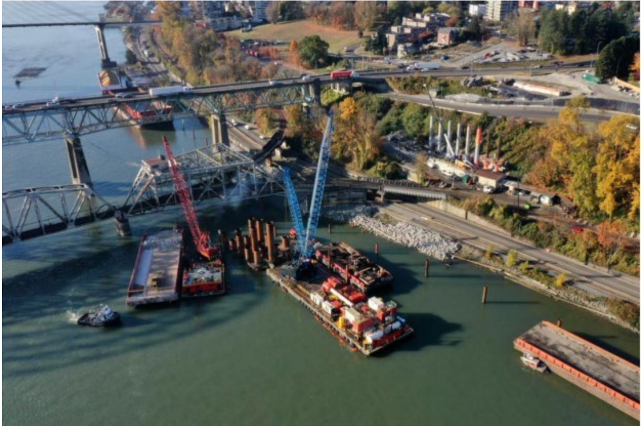
FIGURE 3 – PIER N1 FOUNDATION PILING
