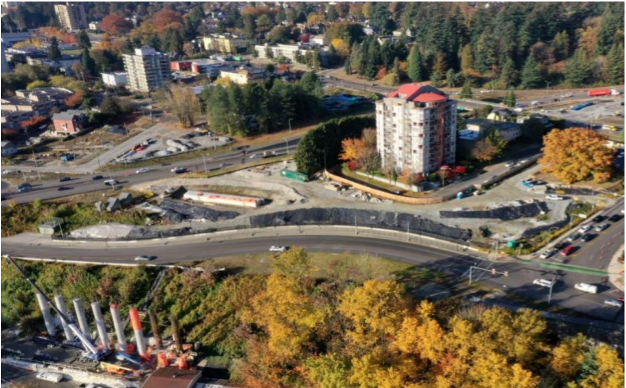
FIGURE 2 – N2 COLUMN CONSTRUCTION (BOTTOM LEFT) AND THE N3 ABUTMENT (MIDDLE LEFT)
