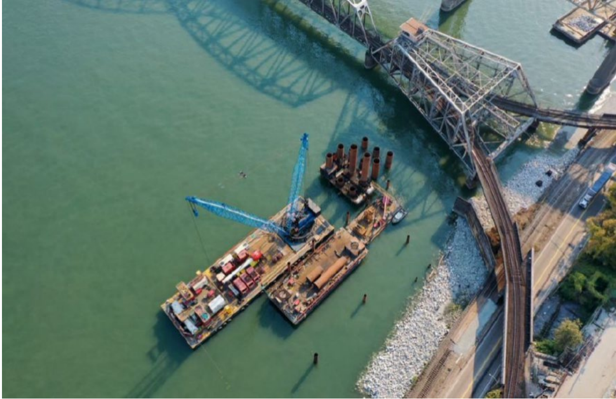
FIGURE 3 – PIER N1 FOUNDATION PILING
