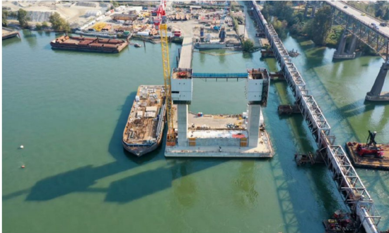
FIGURE 2 – PIER S1 TOWER CONSTRUCTION
