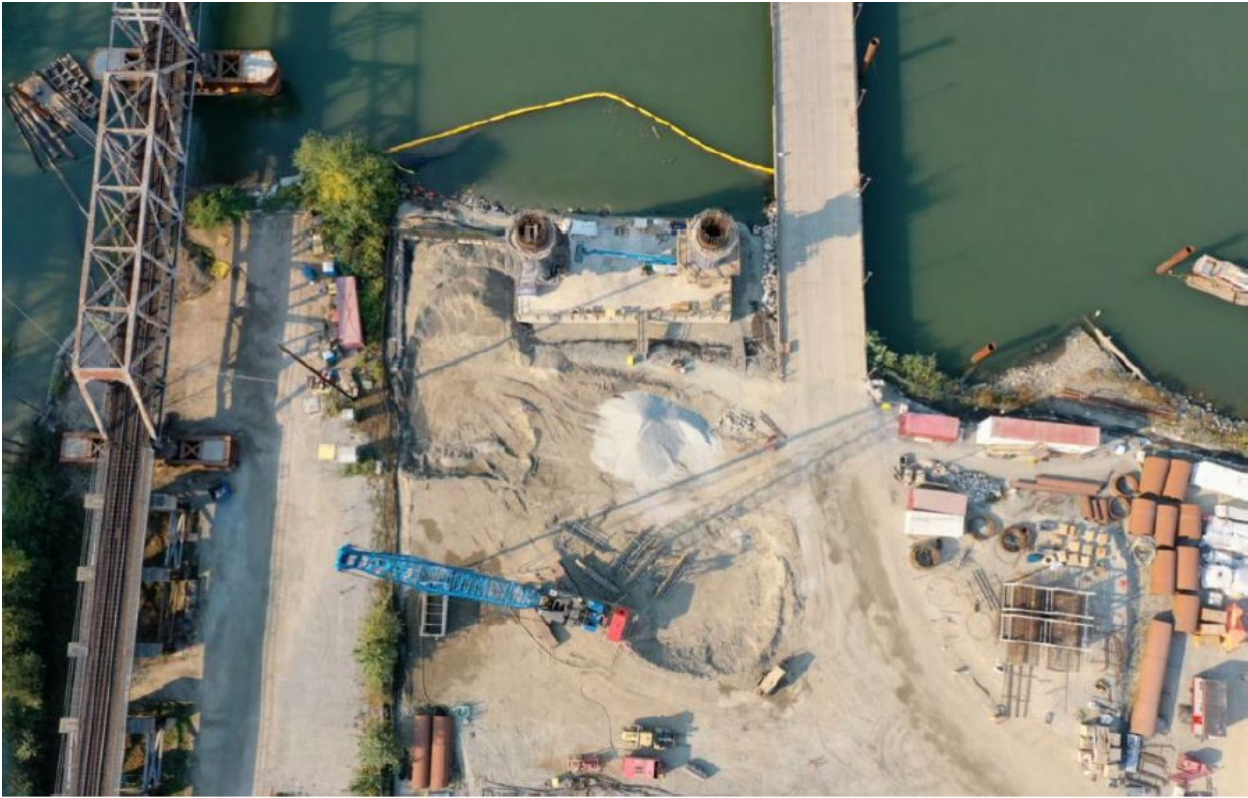
FIGURE 1 – PIER S2 PILE CAP WORK
