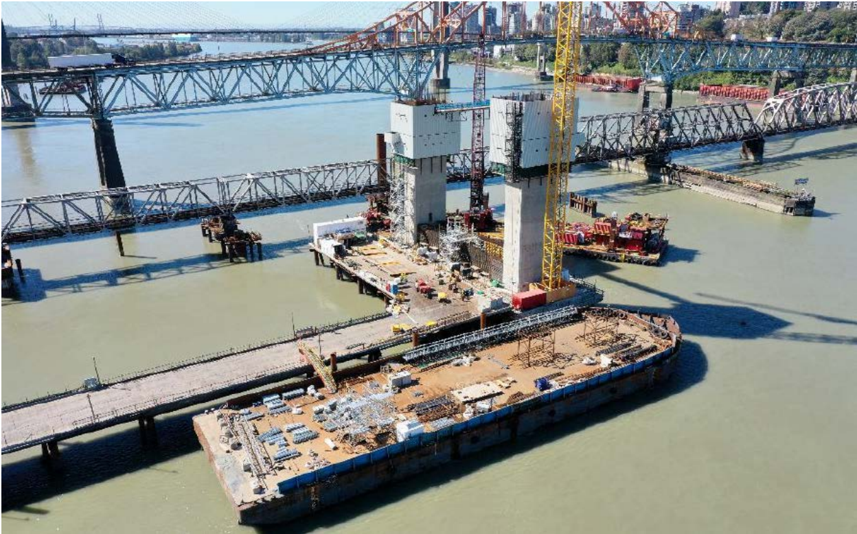
FIGURE 2 –PROGRESS OF THE PIER S1 TOWER CONSTRUCTION
