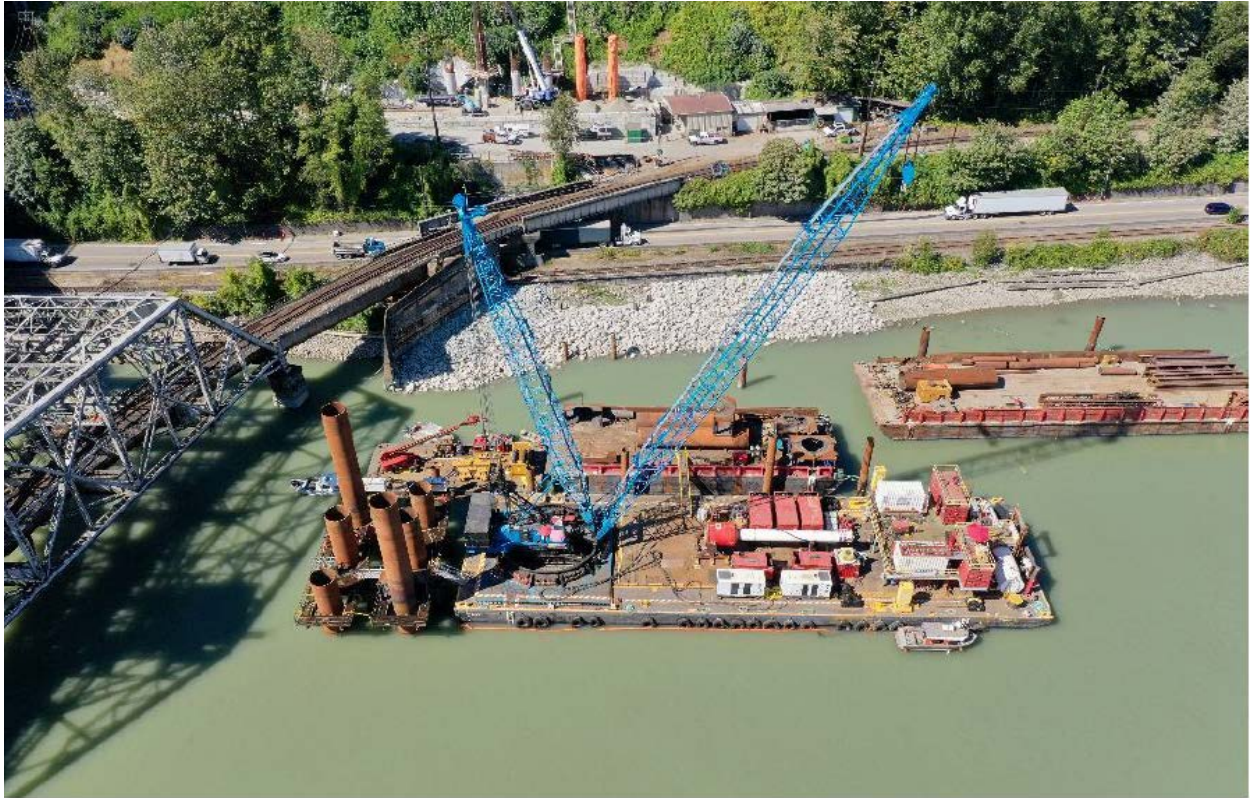
FIGURE 3 – PIER N1 FOUNDATION PILING (FRONT) AND PIER N2 COLUMN CONSTRUCTION (BACK)
