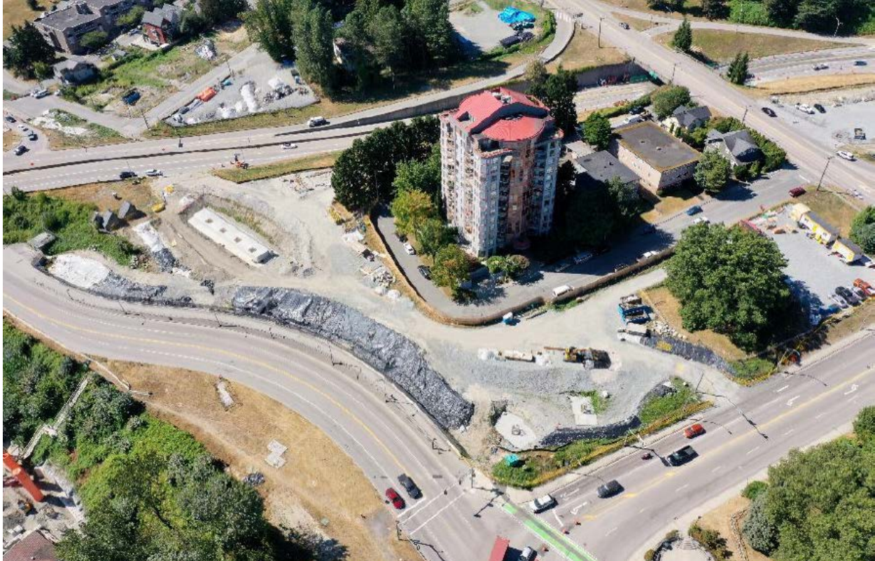
FIGURE 4 – PIER N3 ABUTMENT WORK
