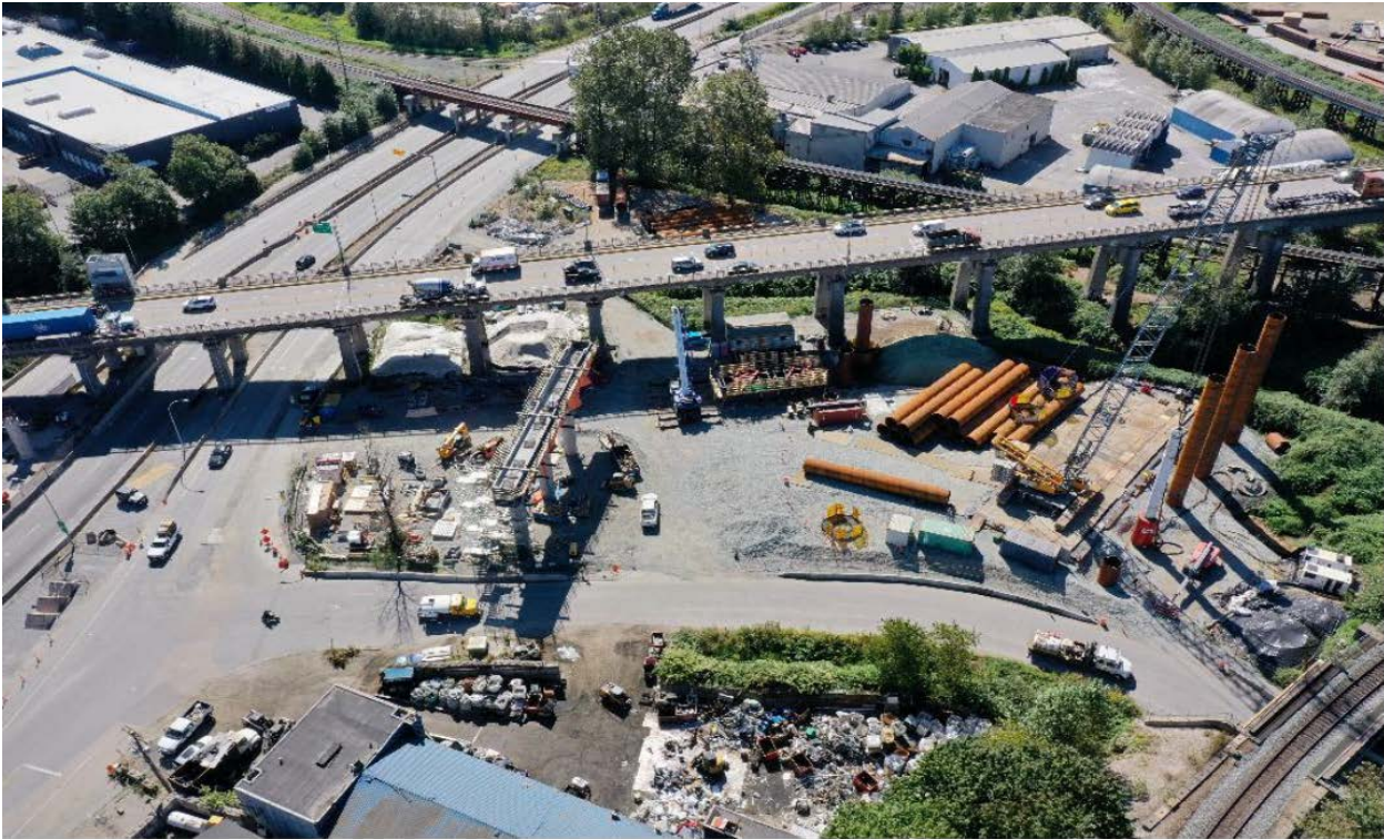
FIGURE 1 –PIER S6 PILE INSTALLATION (RIGHT) AND PIER S7 COLUMNS (LEFT)
