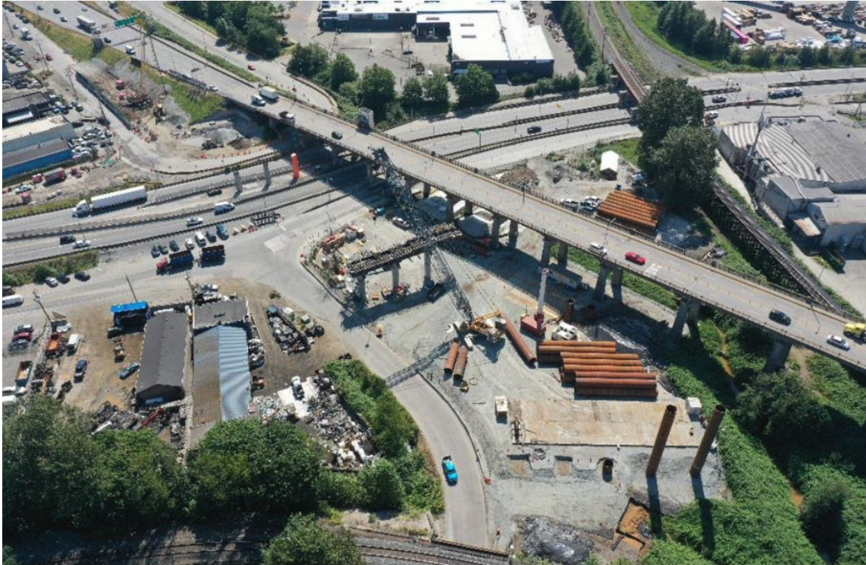
FIGURE 3 – PROGRESS OF THE S6 PILE INSTALLATION AND THE S7 COLUMNS CONSTRUCTION
