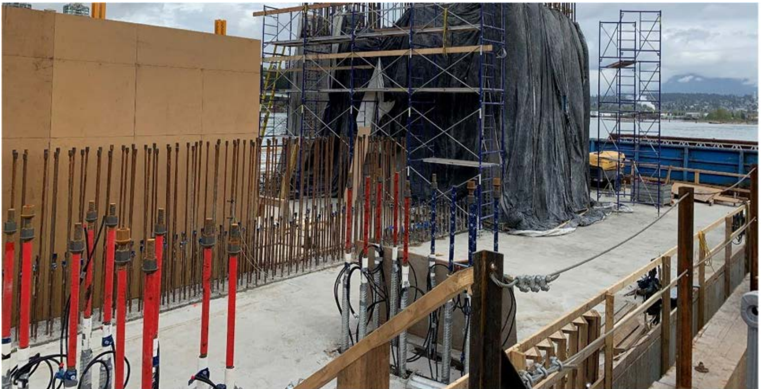
FIGURE 2 – PIER S1 TOWER LEG CONSTRUCTION
