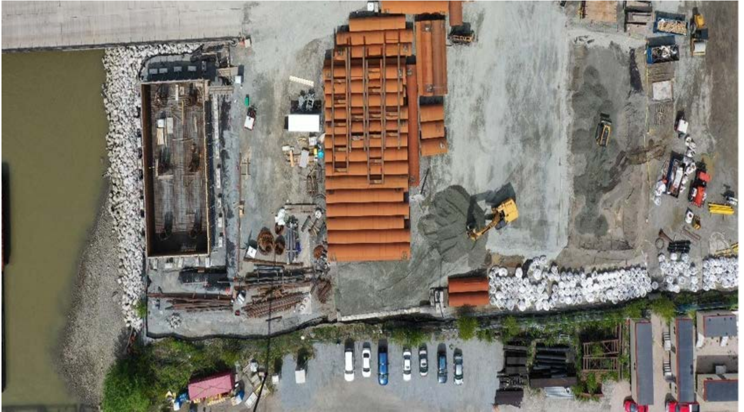
FIGURE 3 – PILE CAP INSTALLATION WORK AT PIER S2 IN SURREY, B.C.
