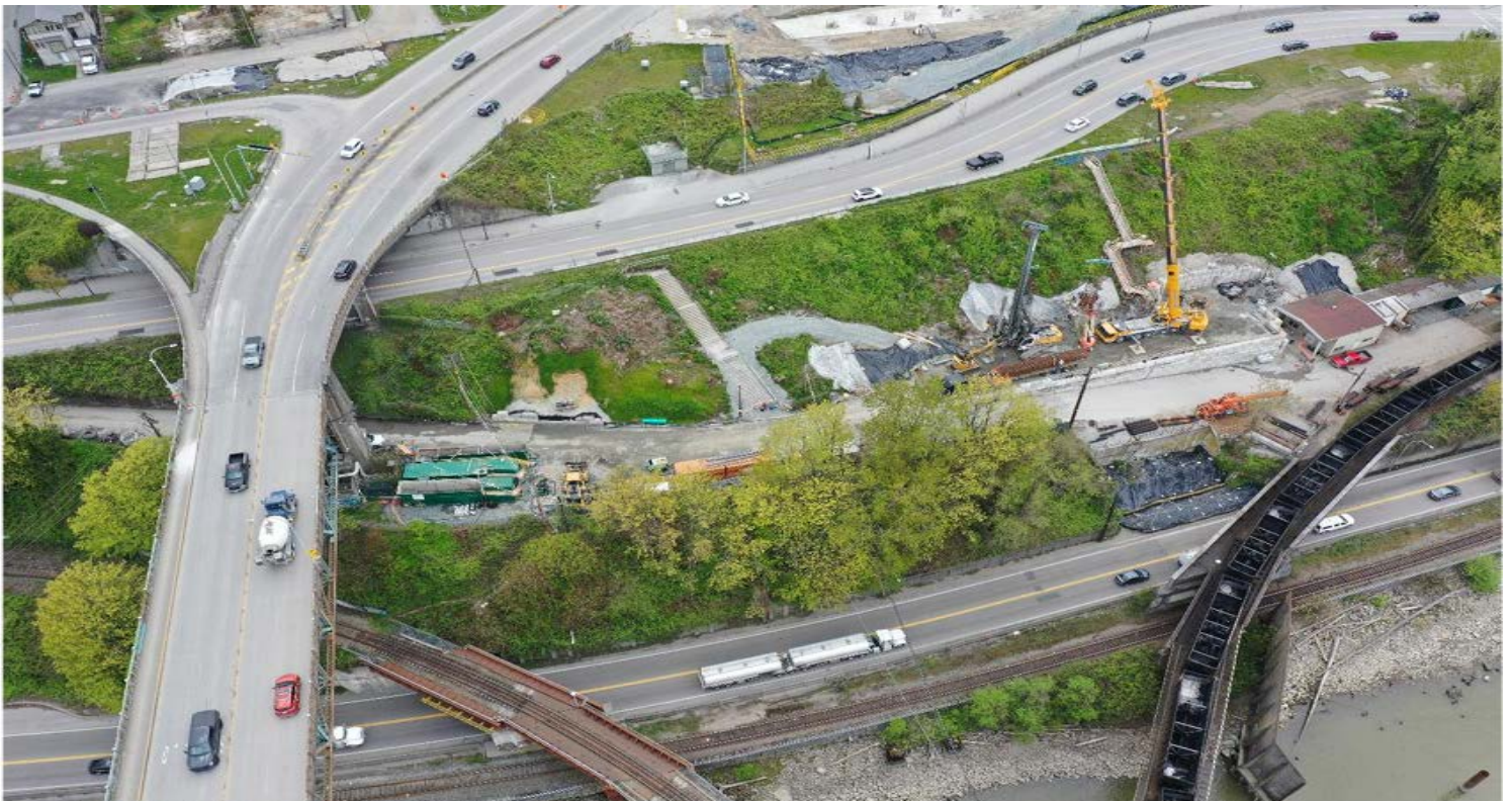
FIGURE 4 – DRILLED SHAFT WORK AREA AT PIER N2 IN NEW WESTMINSTER, B.C.
