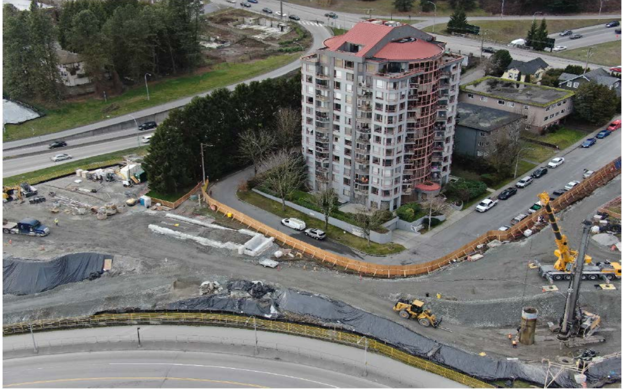
FIGURE 4 – DRILLED SHAFT WORK AREA AT PIER N3 IN NEW WESTMINSTER, B.C.
