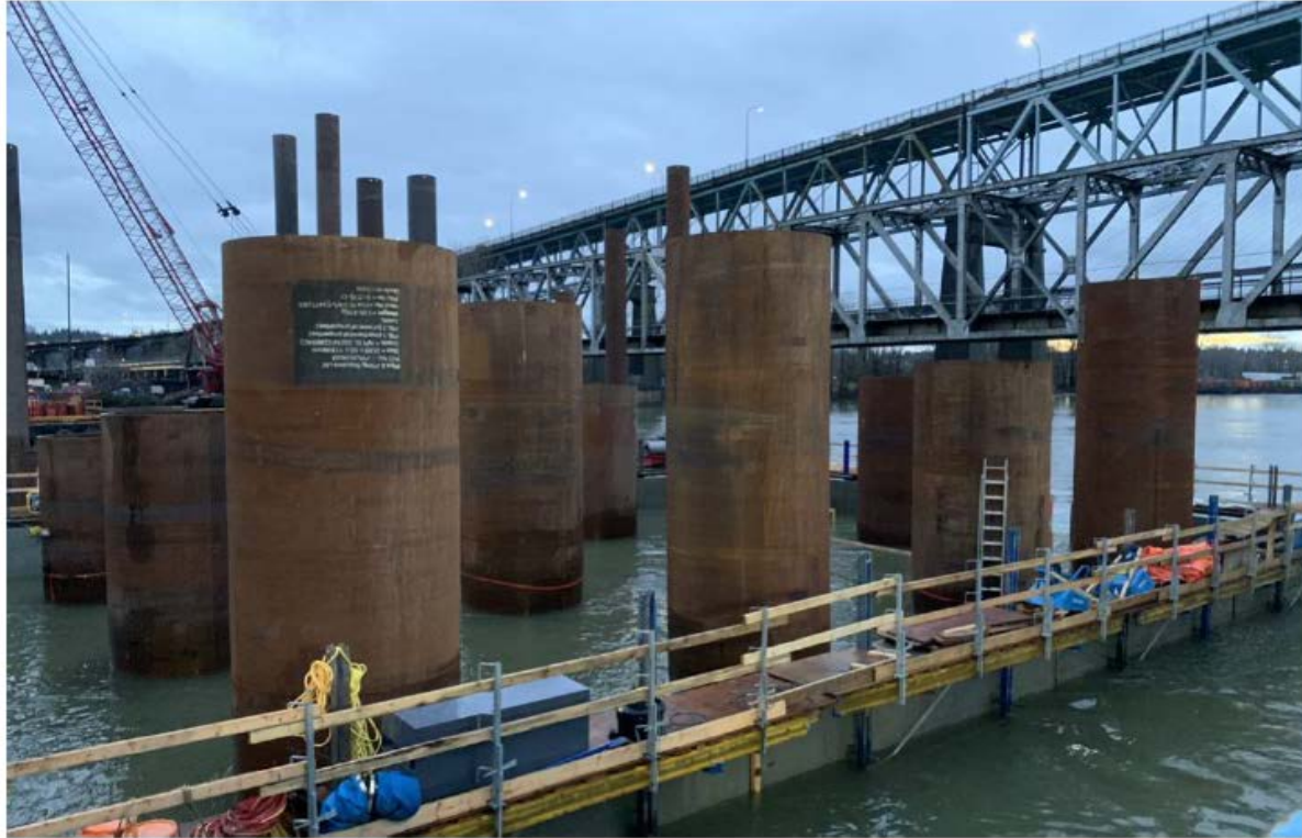
FIGURE 2 –INSTALLATION OF COLLARS AND PRECAST SHELL AT PIER S1
