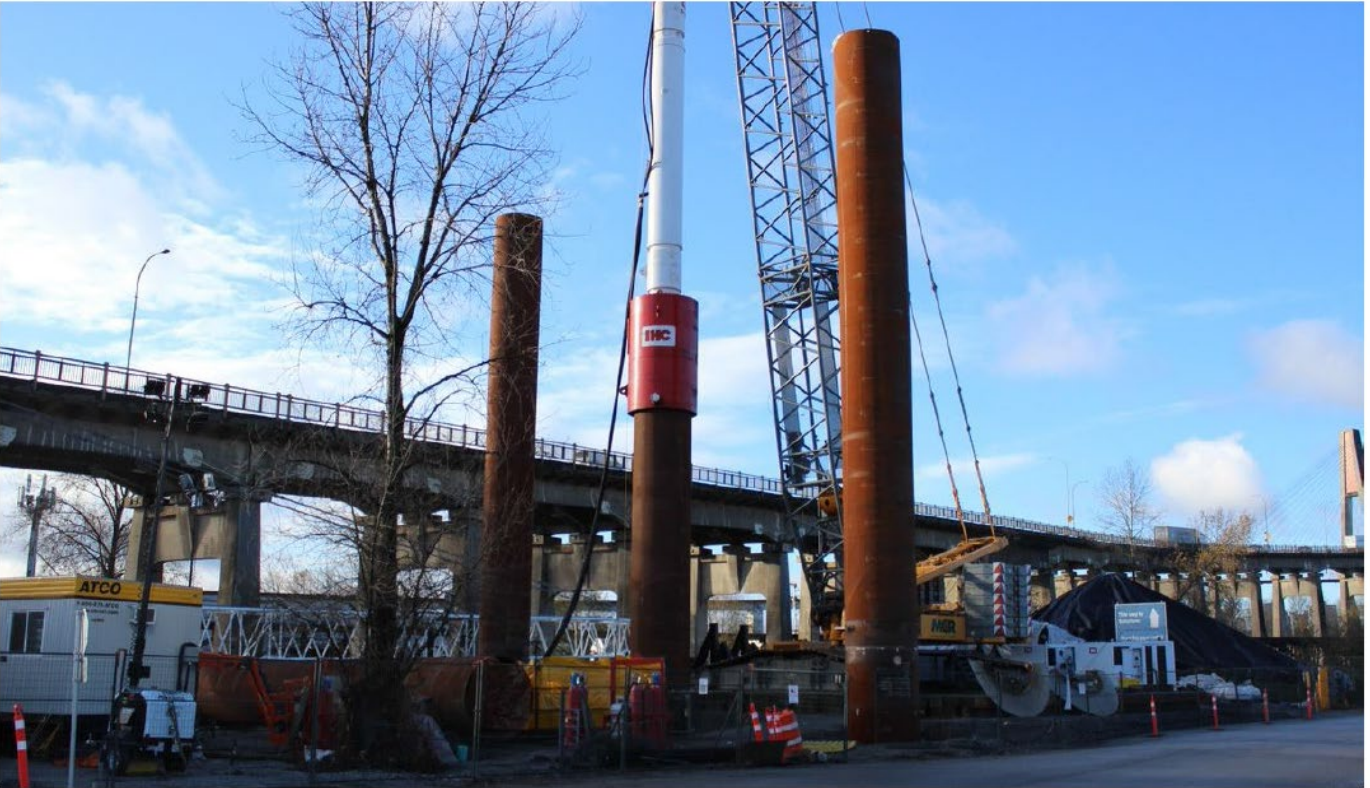
FIGURE 4 – PILE INSTALLATION AT PIER S7
