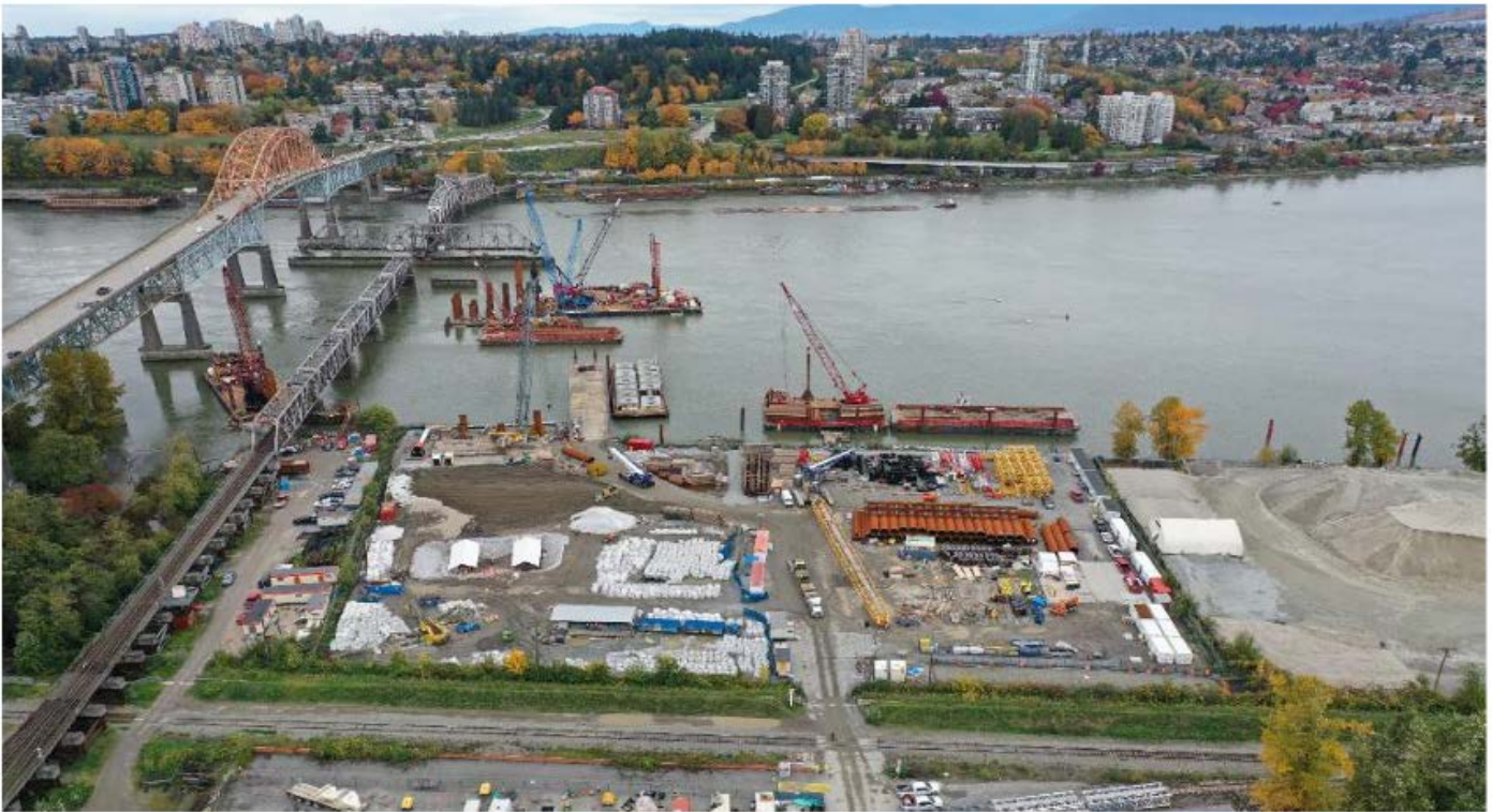
FIGURE 1 – PILE INSTALLATION AT PIERS S1 (BACK) AND S2
