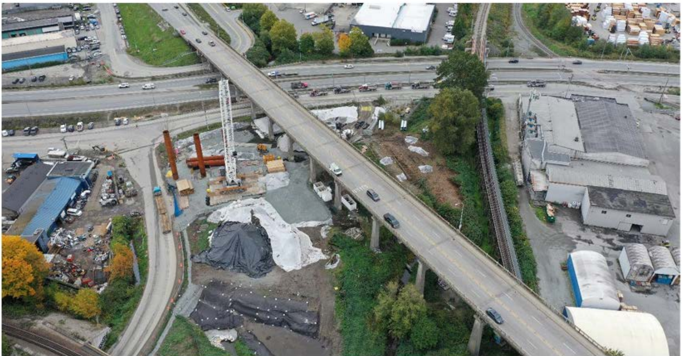
FIGURE 2 – PILE INSTALLATION AT PIER S7
