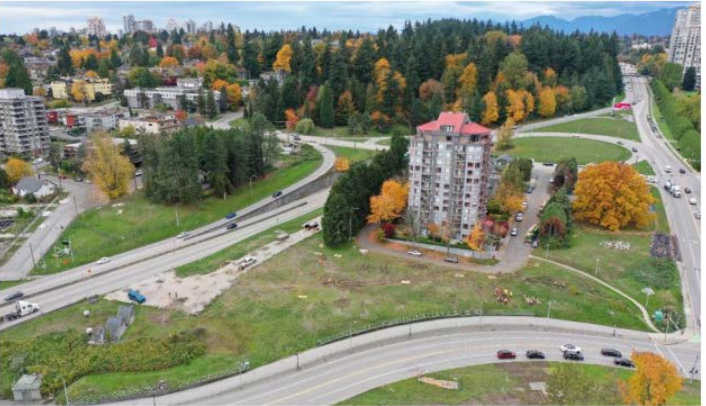
FIGURE 4 – WORK AREA SET UP AT PIER N3 IN NEW WESTMINSTER
