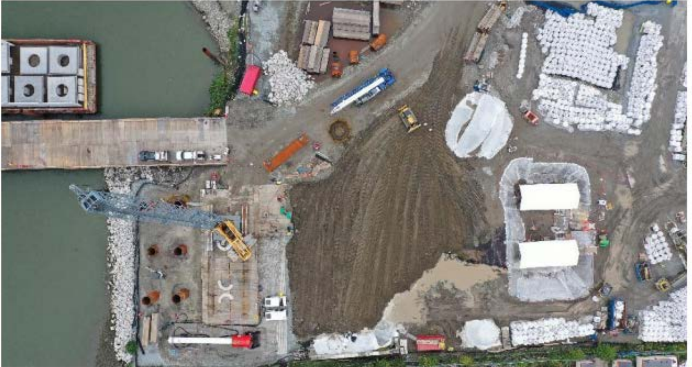
FIGURE 3 – PILE INSTALLATION AT PIER S2 (BOTTOM LEFT)
