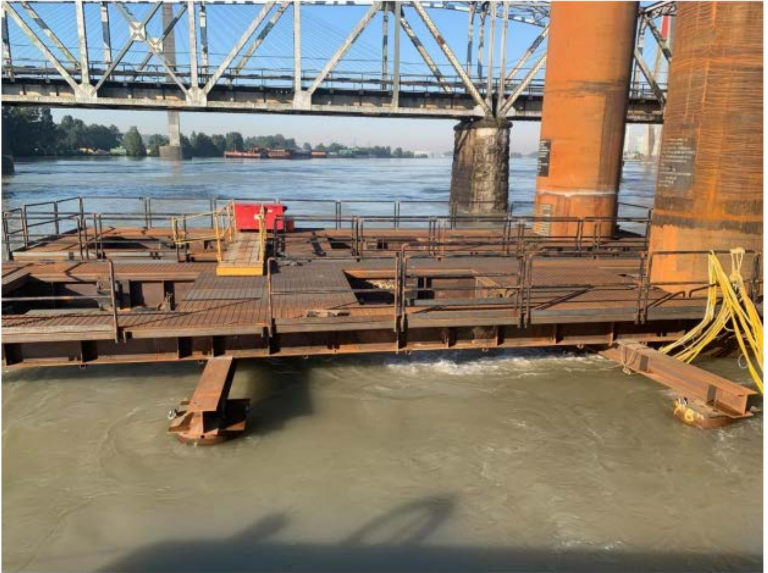
FIGURE 1 – FRAME INSTALLATION ON PIER S1 - PILES 1 AND 4
