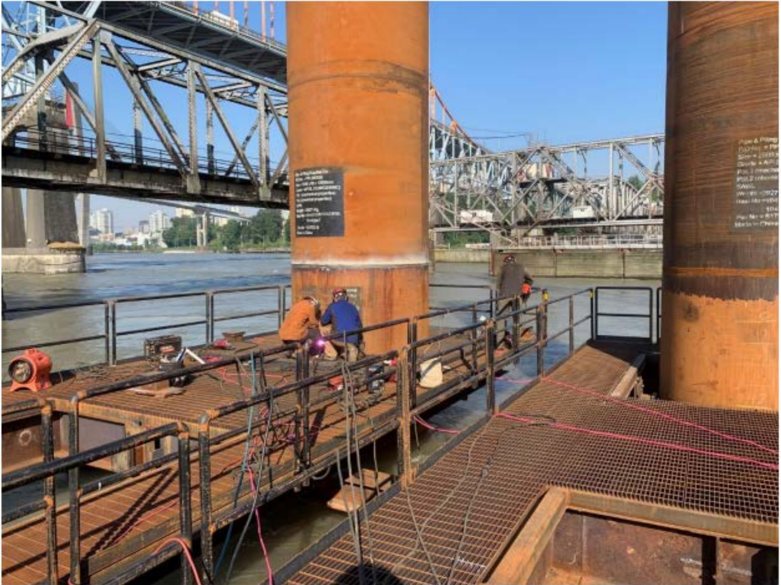
FIGURE 2 – PIER S1 - PILES 1 AND 4 WITH WELDED TOP SECTIONS.
