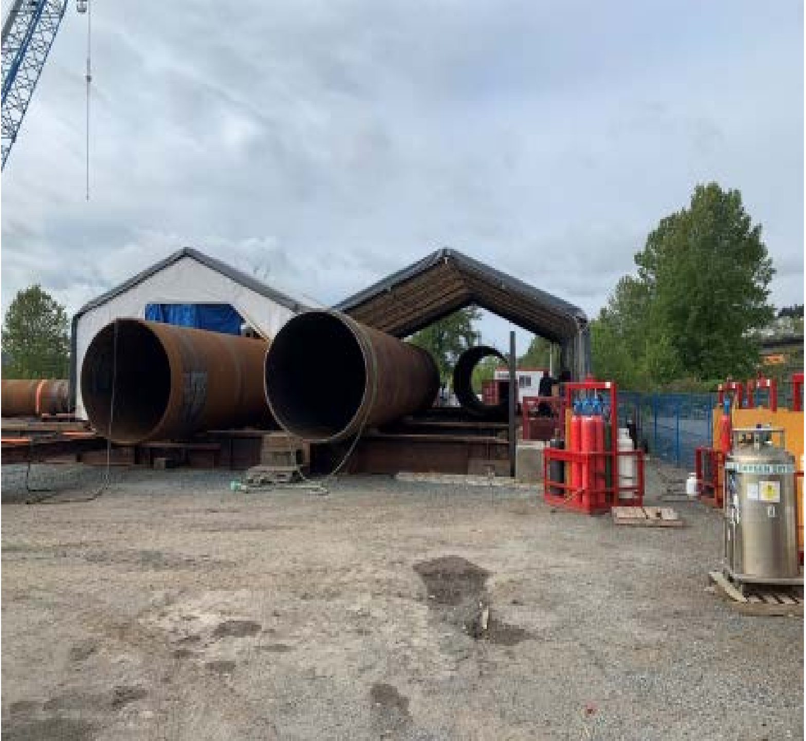
FIGURE 2 –PILE SECTIONS BEING SPLICED AT SPRUCE STREET
