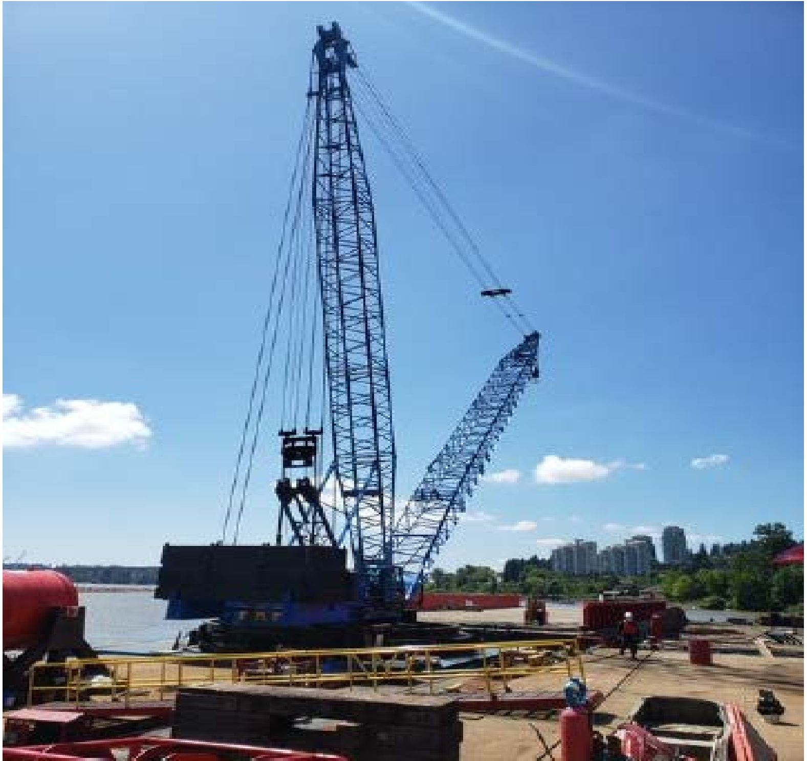
FIGURE 1 – RINGER CRANE SETUP AT SPRUCE STREET YARD
