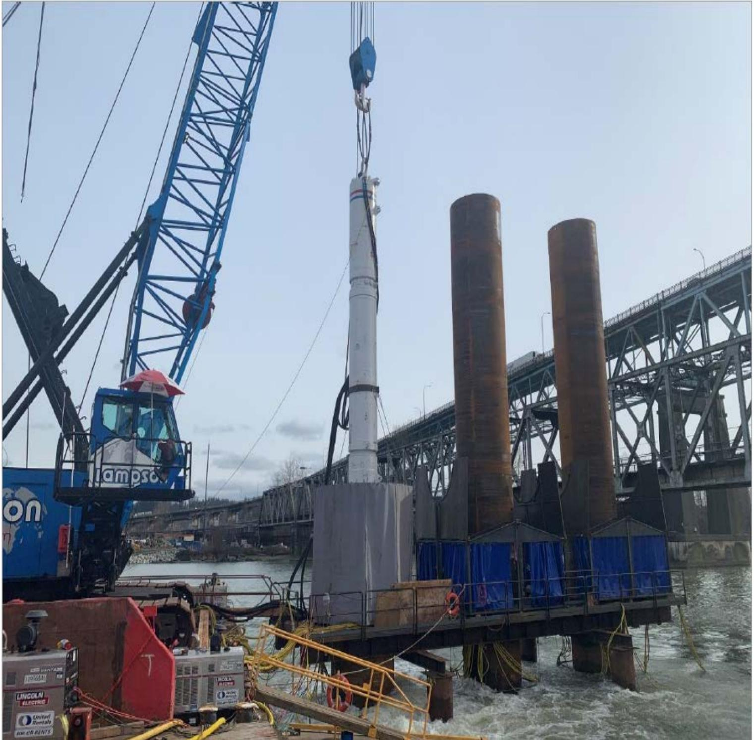
**FIGURE 1 – PILE DRIVING AT S1**
