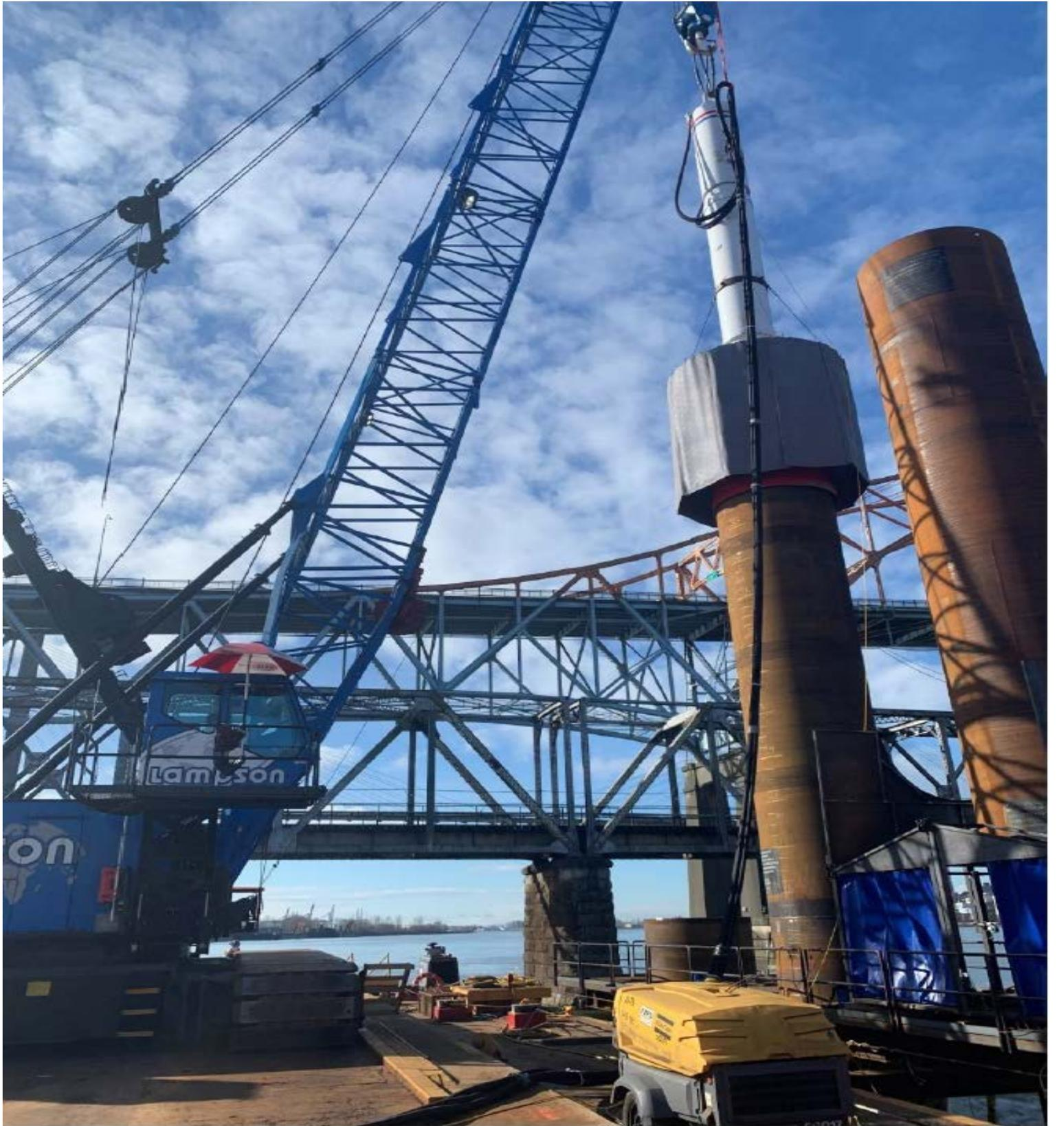
**FIGURE 2 – PILE DRIVING AT S1**
