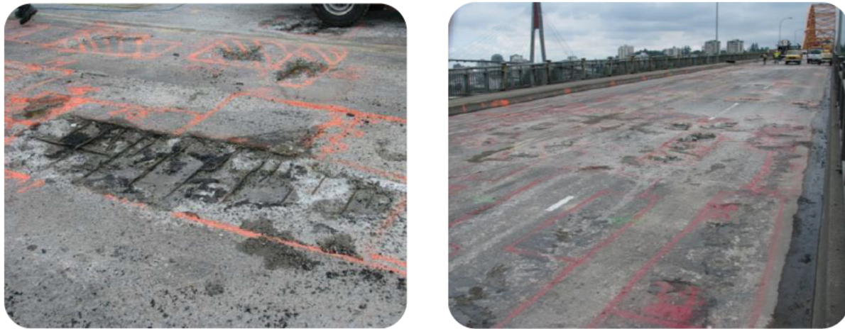
Figure 7: Pattullo Bridge Deck Condition Before Repairs
