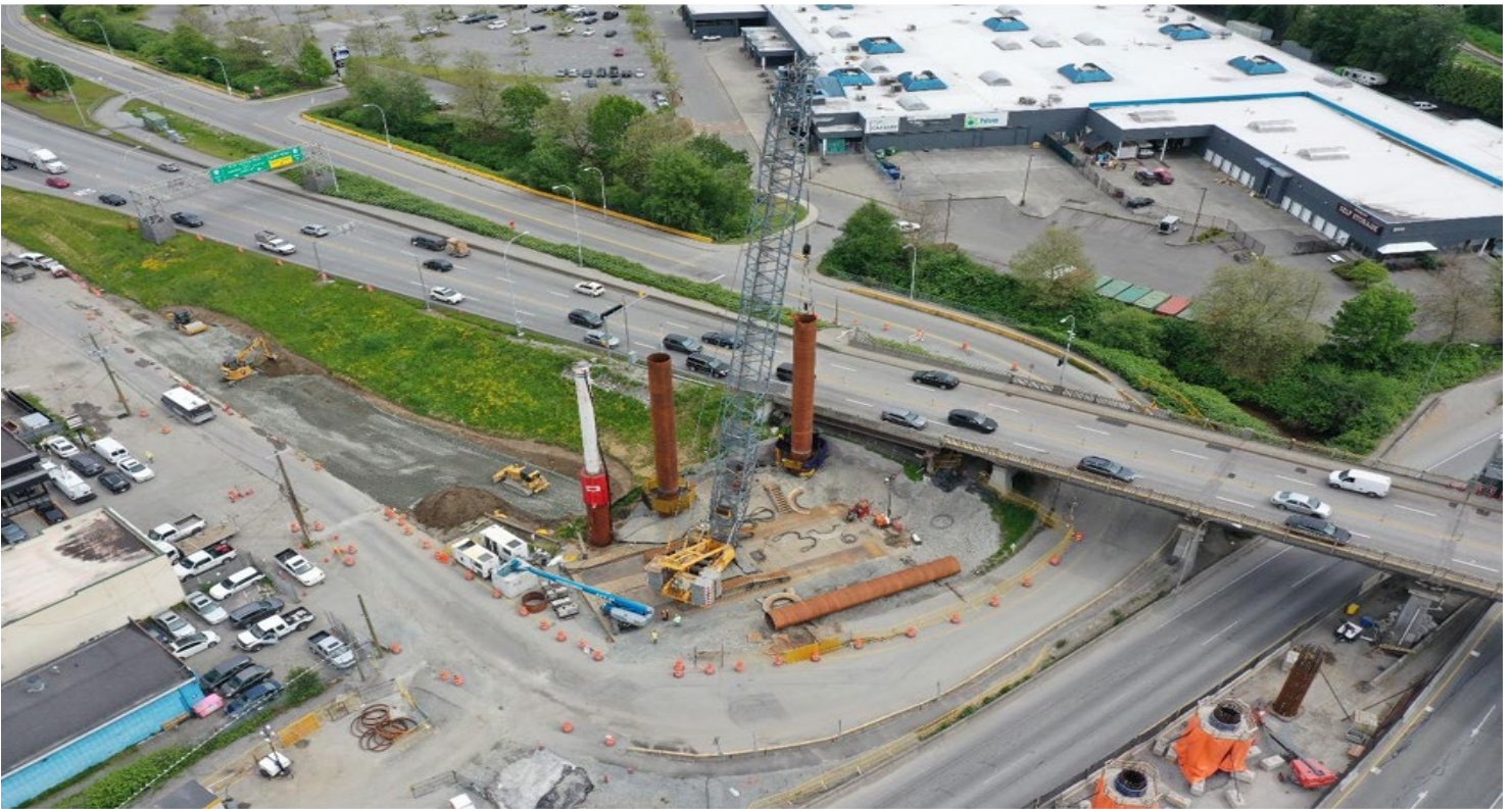
FIGURE 4 – PILE INSTALLATION AT THE SOUTH APPROACH IN SURREY, B.C.
