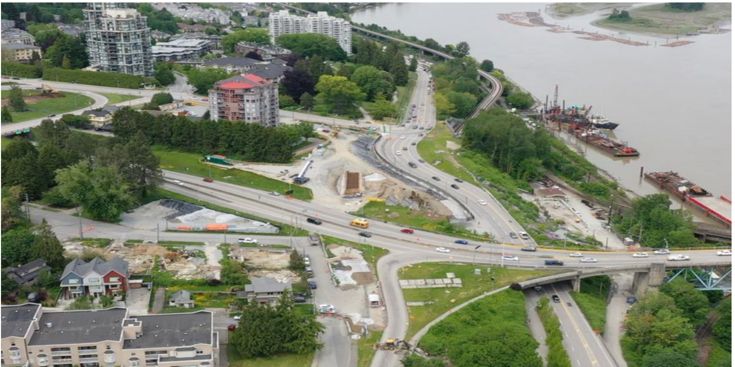
FIGURE 2 – AERIAL SHOWING SITE PREPARATION ACTIVITIES IN NEW WESTMINSTER, B.C.
