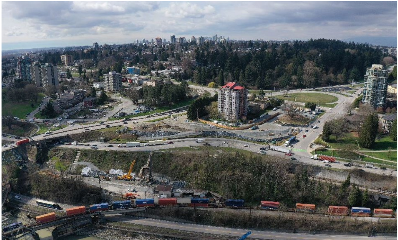
FIGURE 4 – DRILLED SHAFT WORK AREA AT PIERS N2 AND N3 IN NEW WESTMINSTER, B.C.
