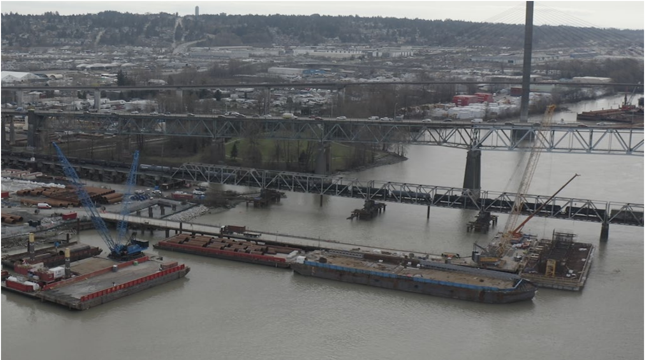
FIGURE 1 – PIER S1 BRIDGE FOUNDATION – PILE PLUG WORK AND REBAR CAGE SETTING COMPLETE
