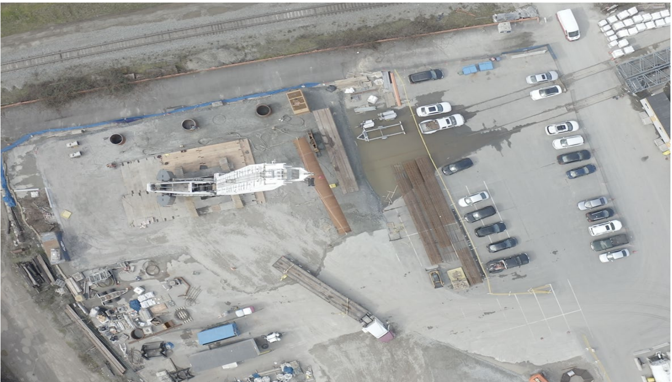
FIGURE 2 – PILE INSTALLATION AT PIER S4 IN SURREY, B.C.
