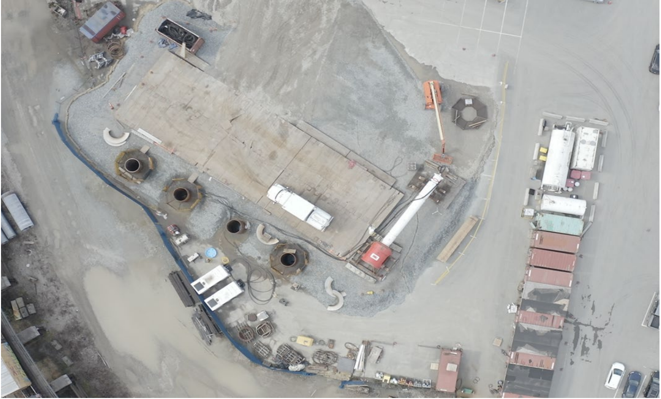
FIGURE 3 – PILE INSTALLATION AT PIER S5 IN SURREY, B.C.
