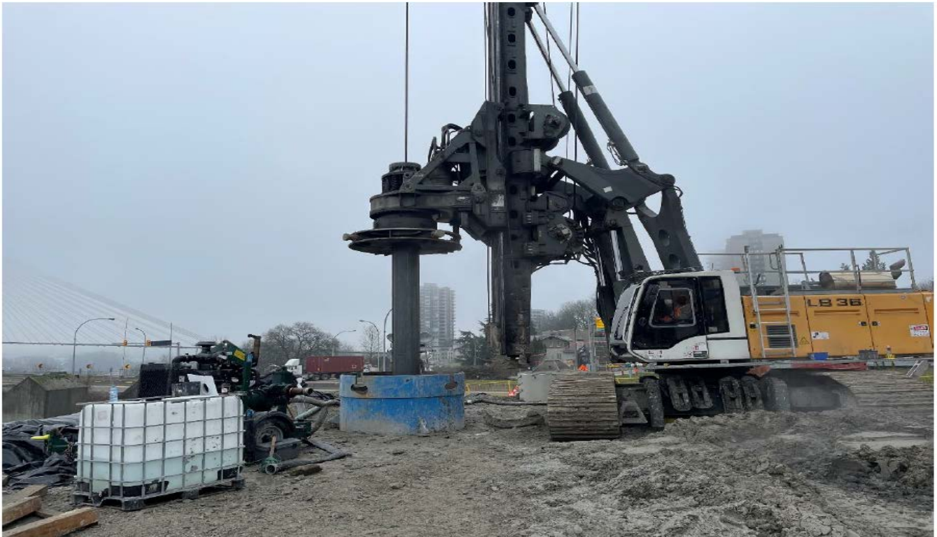
FIGURE 1 – DRILLED SHAFT INSTALLATION AT PIER N3 IN NEW WESTMINSTER, B.C.
