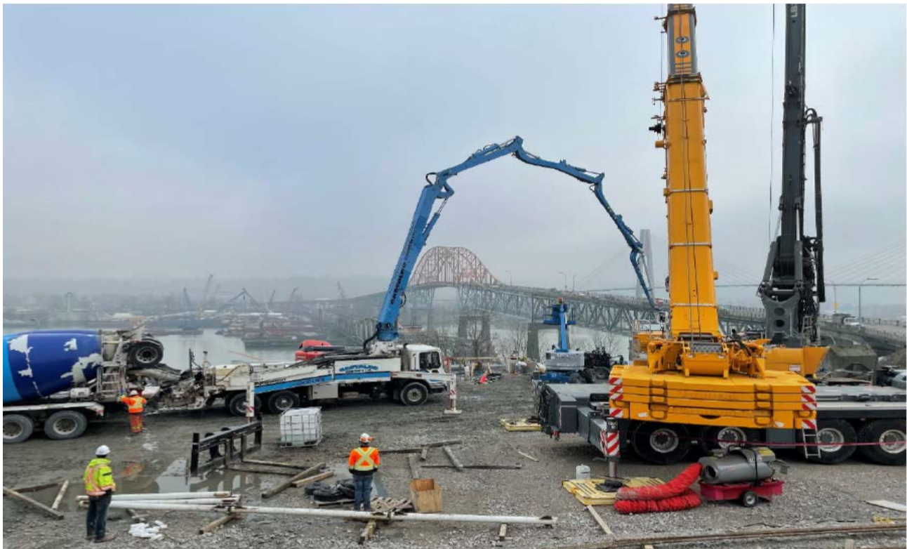
FIGURE 4 – FOUNDATION CONCRETE POURING AT PIER N3 IN NEW WESTMINSTER, B.C.
