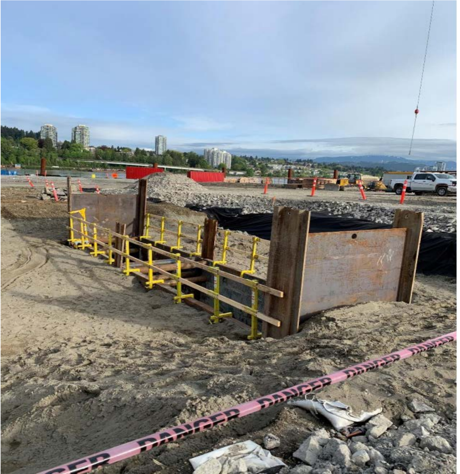
FIGURE 2 – S3 TRENCH BOX FOR ARCHAEOLOGICAL RECOVERY PROGRAM
