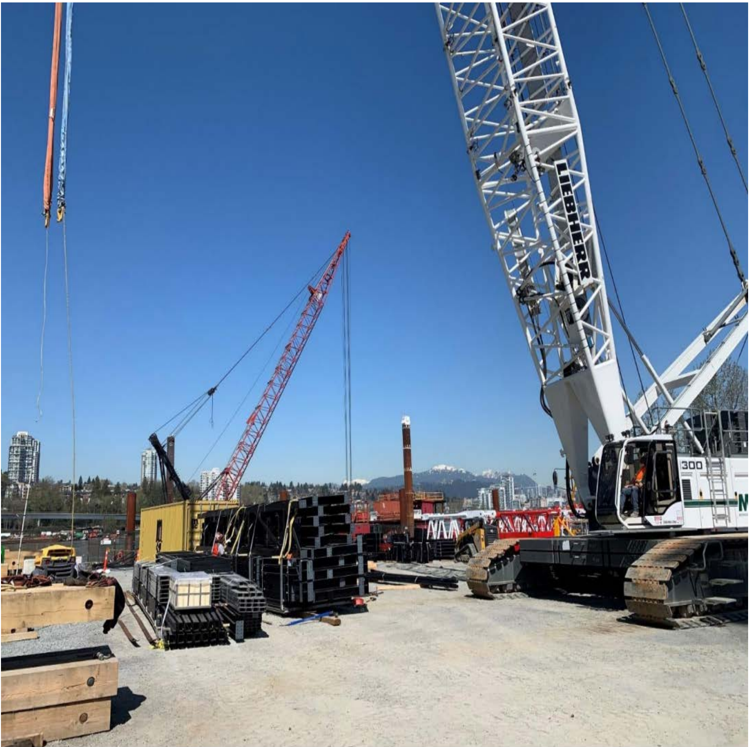
FIGURE 1 – UNLOADING OF THE CLIMBING FORM SYSTEM
