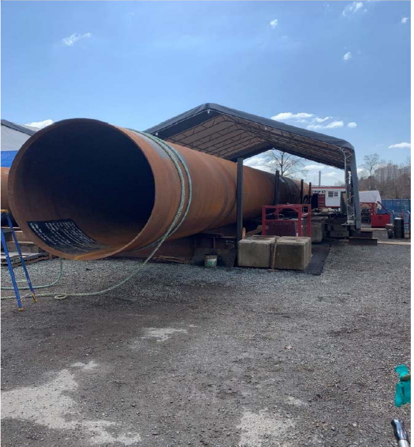
FIGURE 1 – PILE SPLICING OF STARTER SECTIONS
