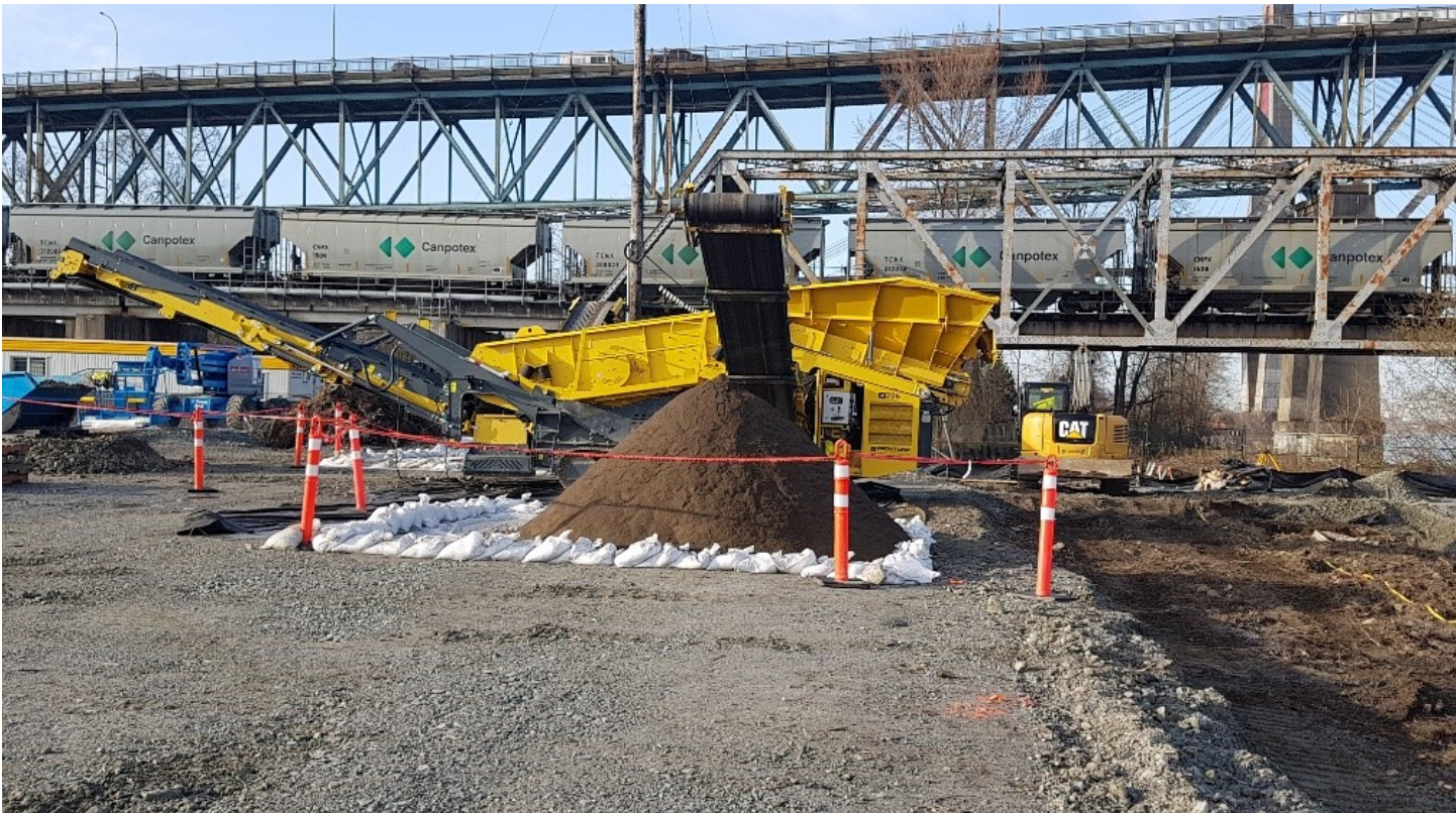
FIGURE 2 – MECHANICAL SCREENER AT S2
