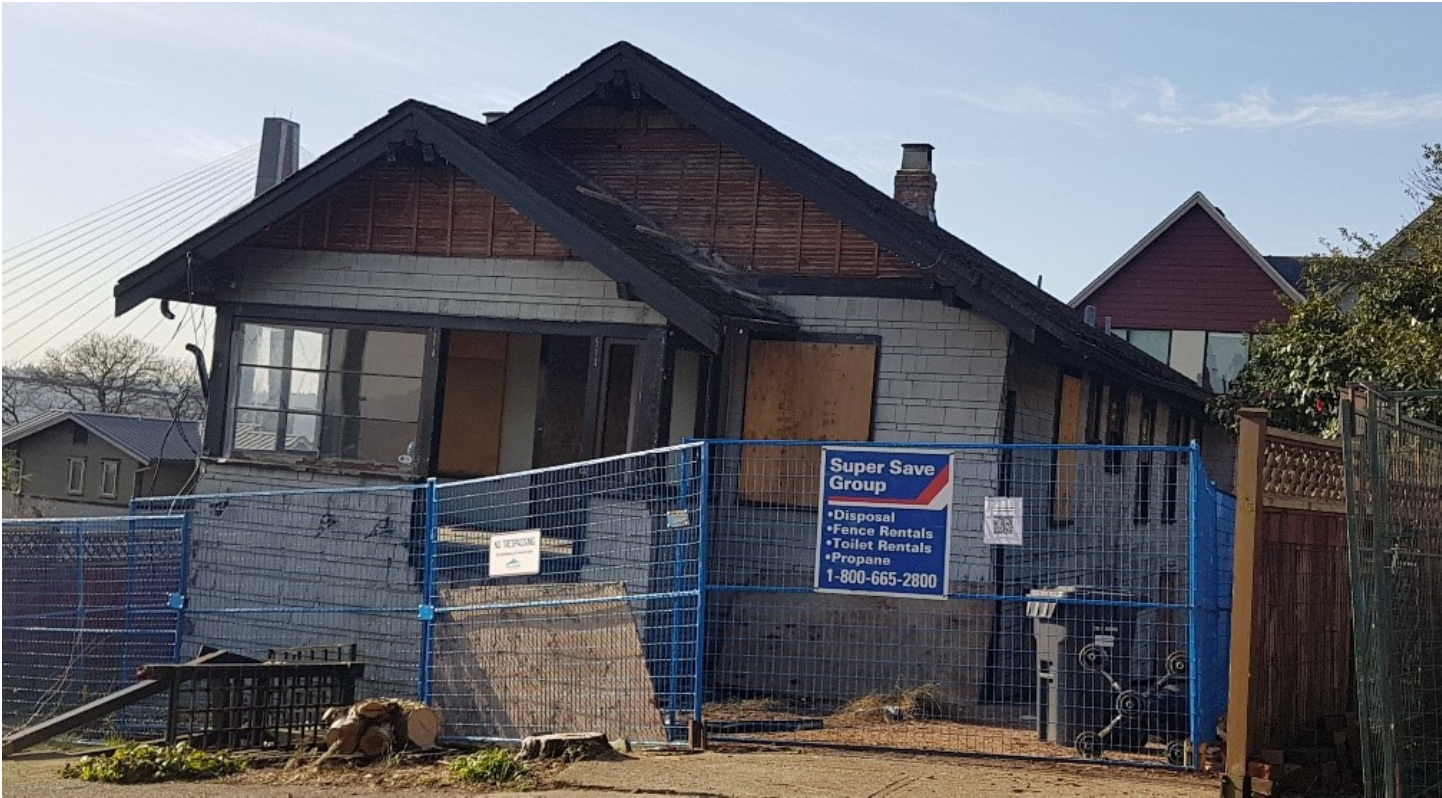
FIGURE 3 – HOUSE DEMOLITION IN NEW WESTMINSTER
